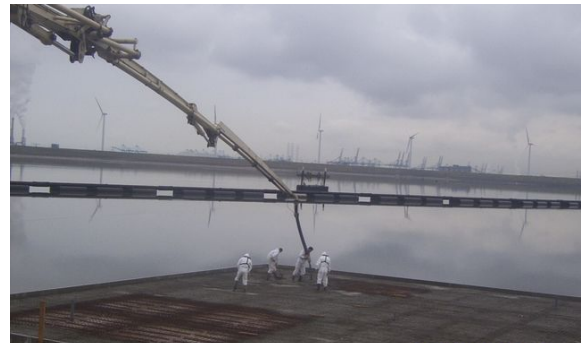
Figure 33: Pouring the concrete floor
