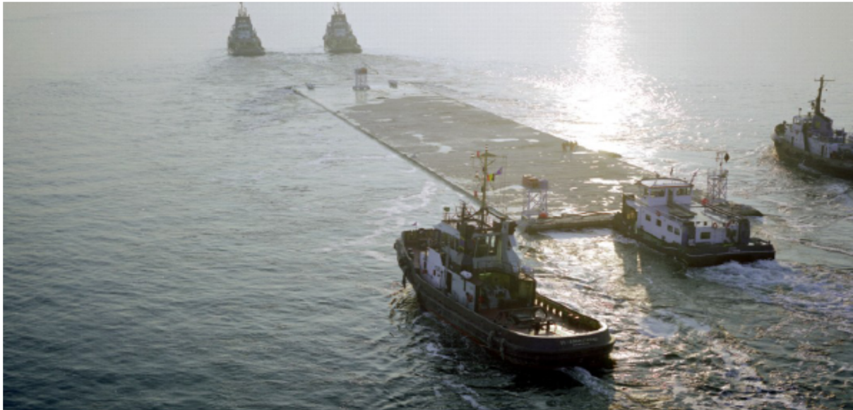
Figure 9: Transport of tunnel element by tugboats, Piet Hein Tunnel [www.bam.nl]
