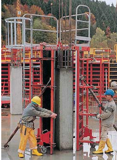
Figure 35: Panel formwork for column [PERI BV]
