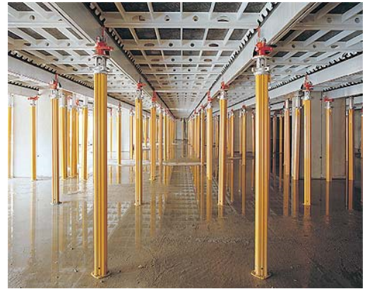
Figure 37: Panel formwork for the roof/floor [PERI BV]
