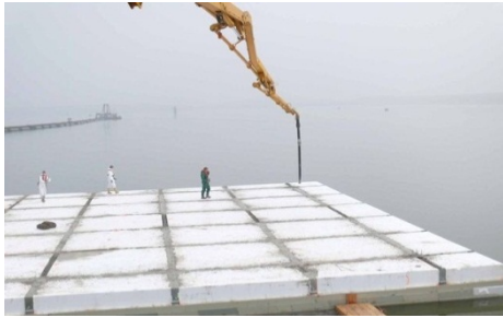
Figure 32: Concrete pump pouring the beam grid
