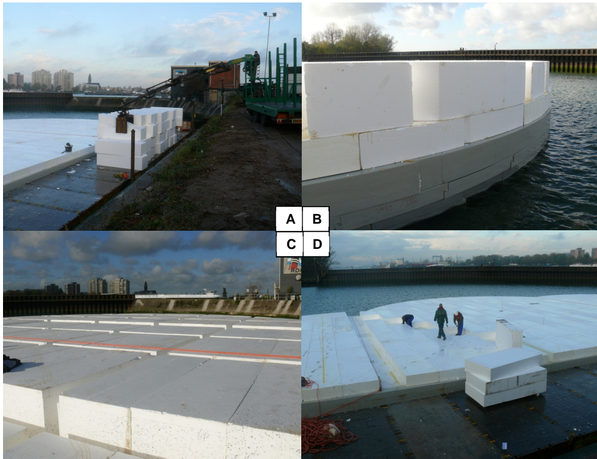
Figure 29: A: Unloading of the EPS blocks C: Top-view EPS formwork
