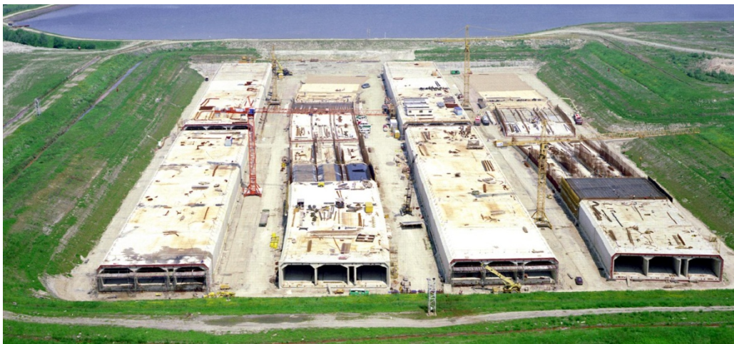
Figure 8: Construction of tunnel elements in dry dock, Piet Hein Tunnel [www.bam.nl]
