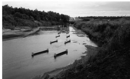
Figure 1-6. Submerged vanes (early version) in East Nishnabotna River, Iowa, protecting stream bank against erosion. View is downstream at extreme low flow, showing vane-induced sediment deposition along right bank. The sediment deposits provide natural toe protection at the bank.
