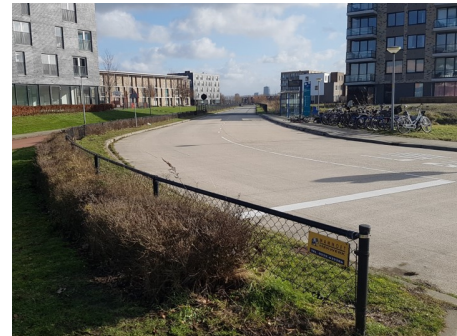
Fig. 3: Segregated bus infrastructure Almere
