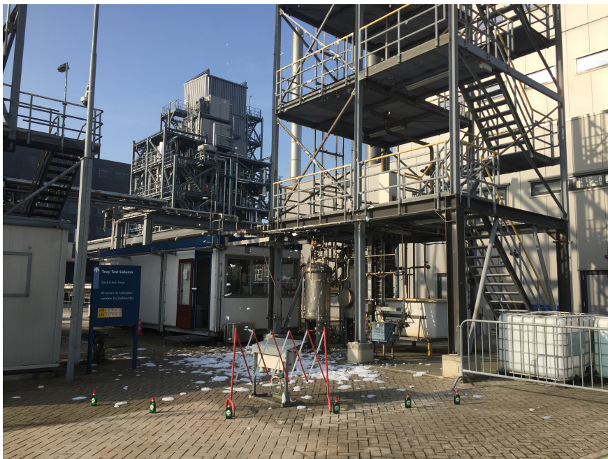
Figure B.12: Foam which is vented to the atmosphere with the air from the separator.
