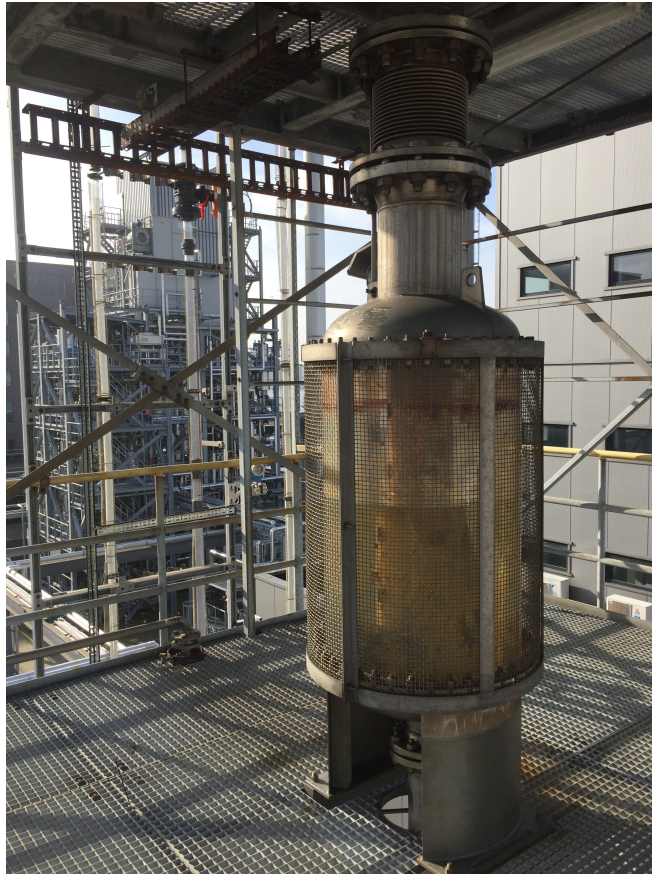
Figure B.1: The separator (V-202).
