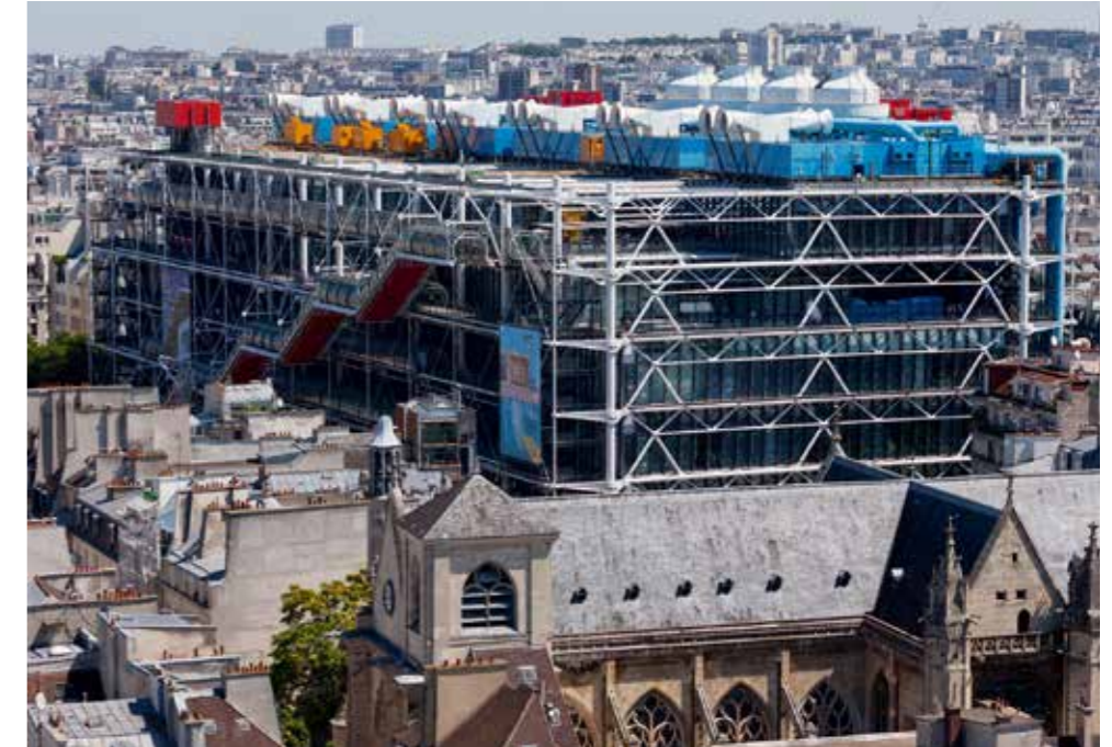
Centre Pompidou | Rogers & Piano
