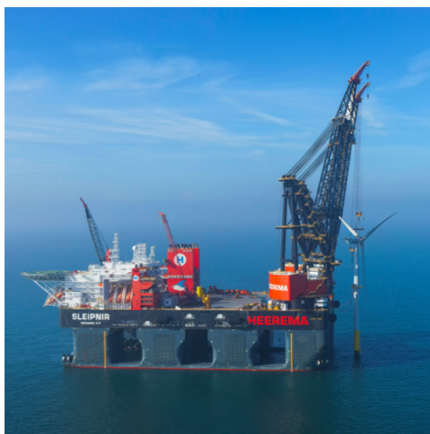
(a) Floating Wind Turbine Installation (TU Delft, 2021)
