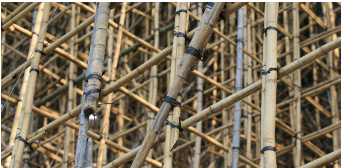
Figure 2.22 Scaffolding rope connection
