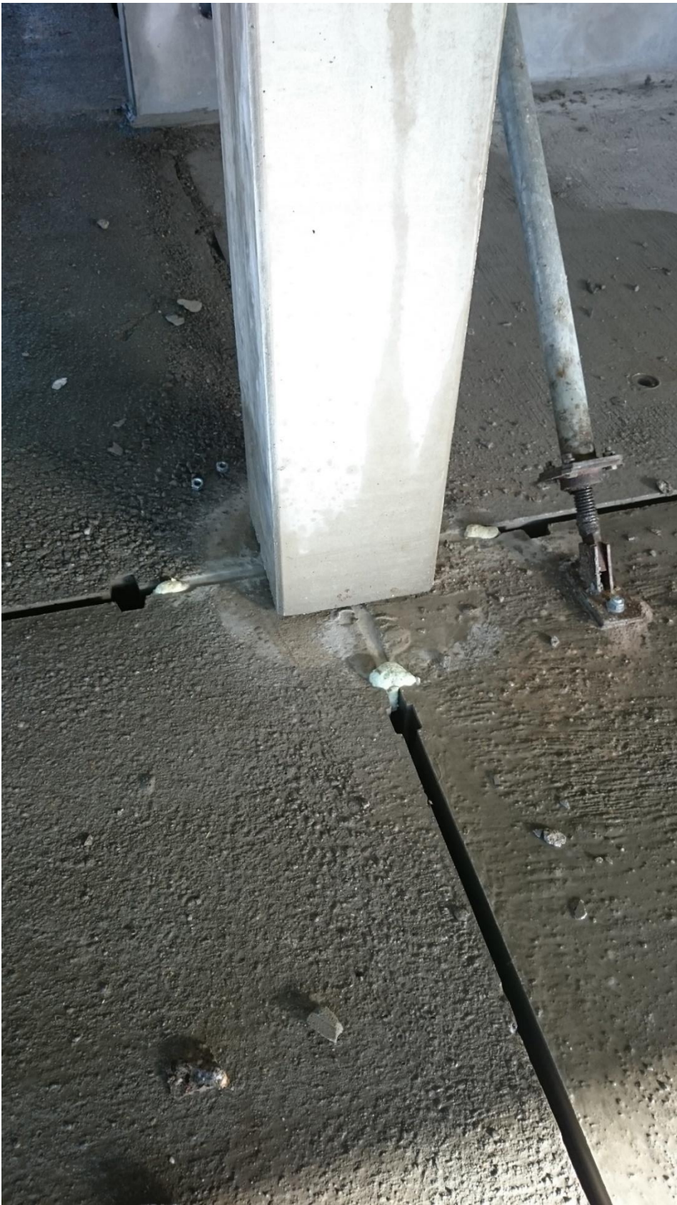
FIGURE 27: COLUMN TO FLOOR CONNECTION, WITH MORTER
