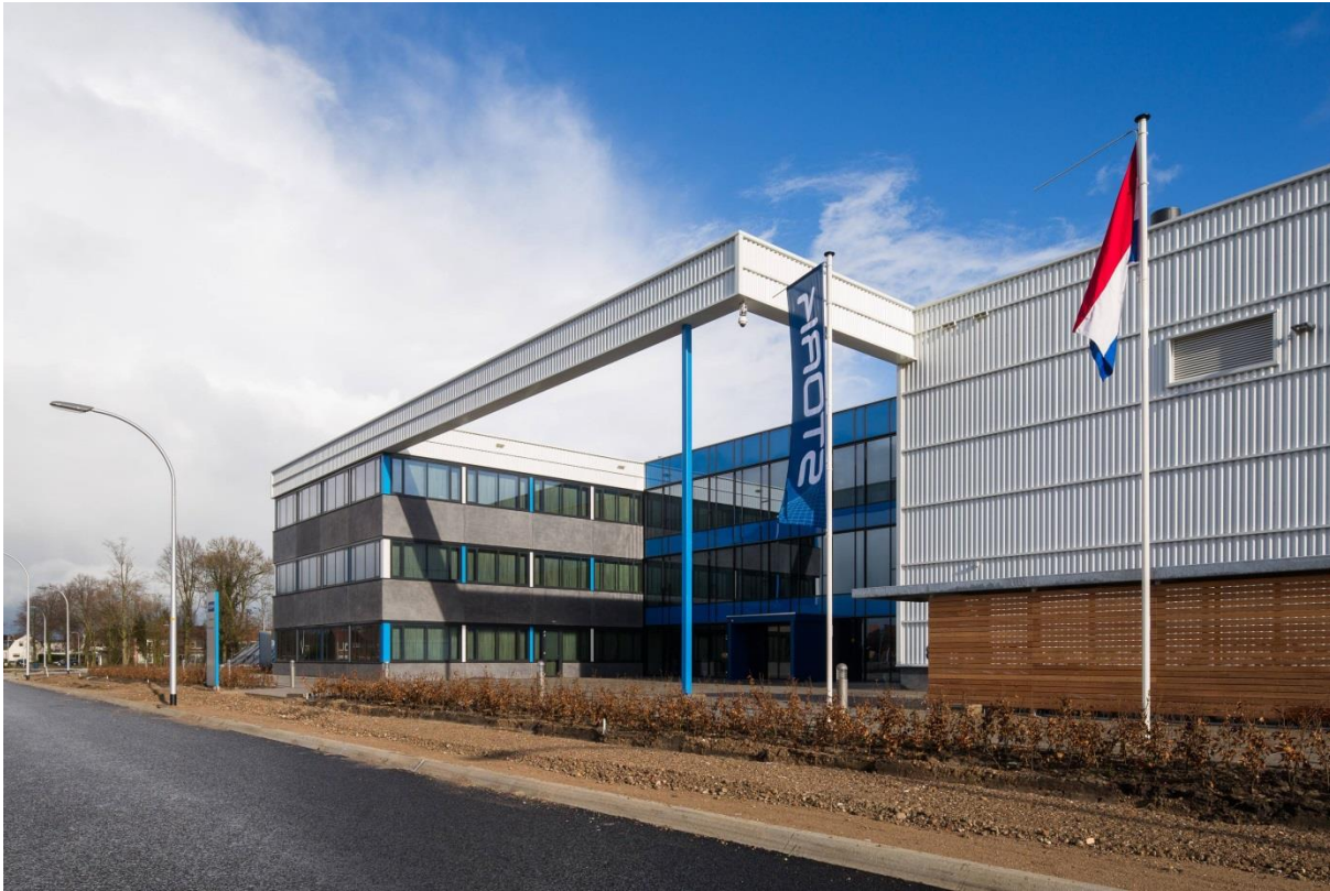
FIGURE 60: PICTURE OF THE REAL BUILDING
