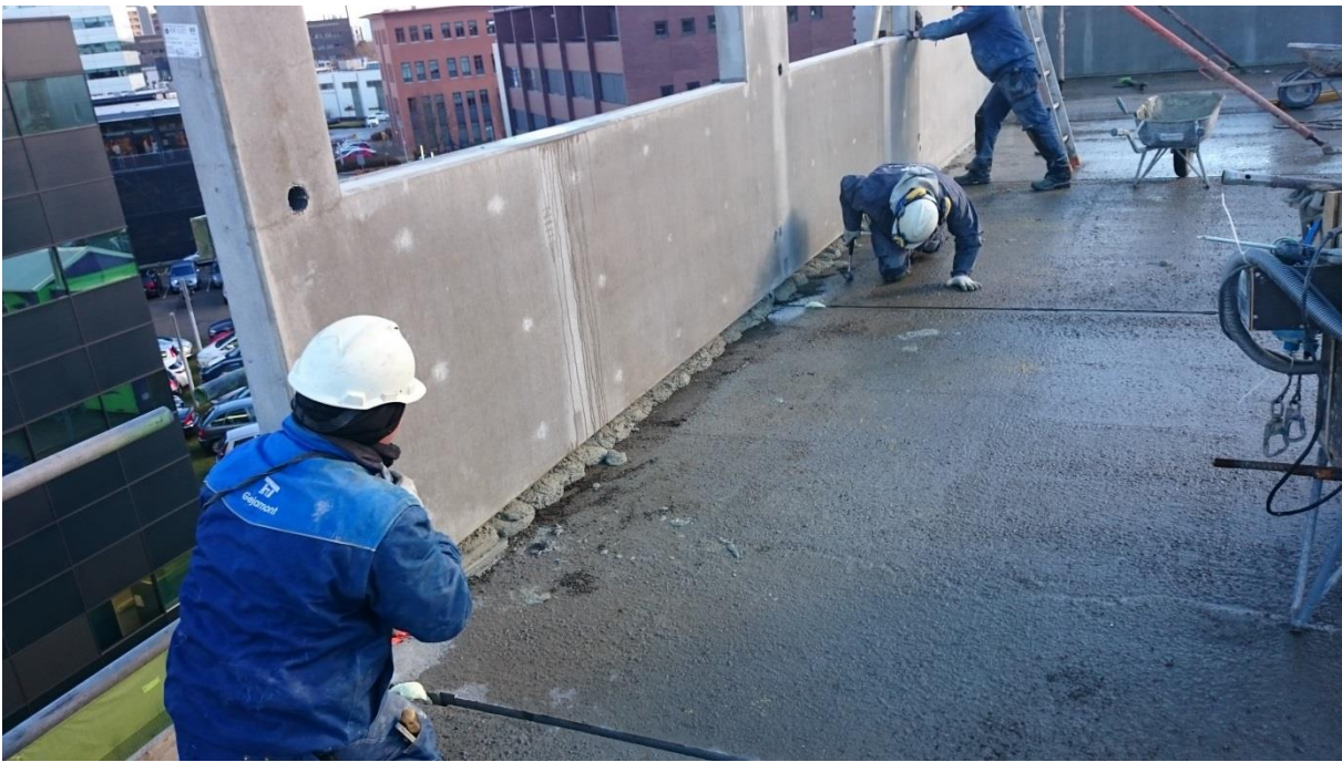
FIGURE 23: PLACING OF A WALL ELEMENT
