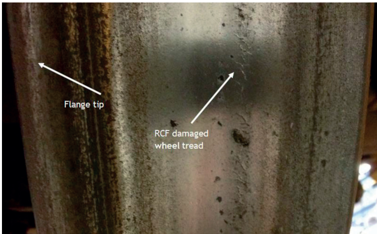
Figure 1. Wheel tread with RCF crack damage.
