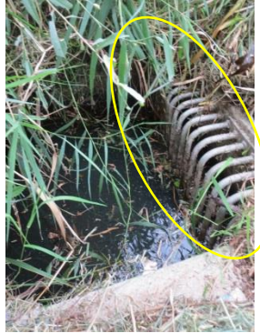
Figure 3.5 View of intake structure (intake circled)
