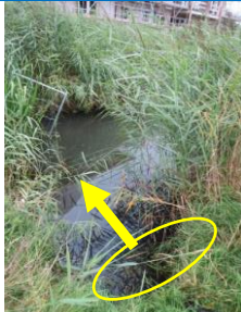
View of cold water discharge area (discharge headwall location indicated by circle, flow direction of cold water indicated by arrow)
