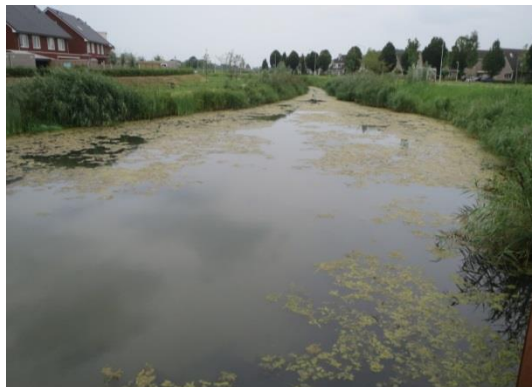
View of channel from bridge near intake, facing east
