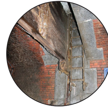
14 old sluice-gate in its construction groove
