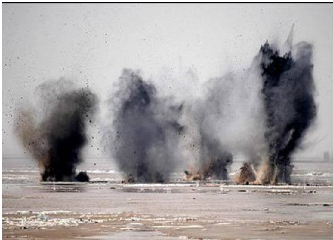
Photo 10 Using bombs to destroy the ice blocks
