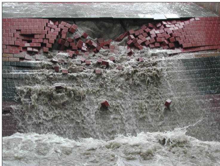
b. Revetment starts to collapse during Test T11C
