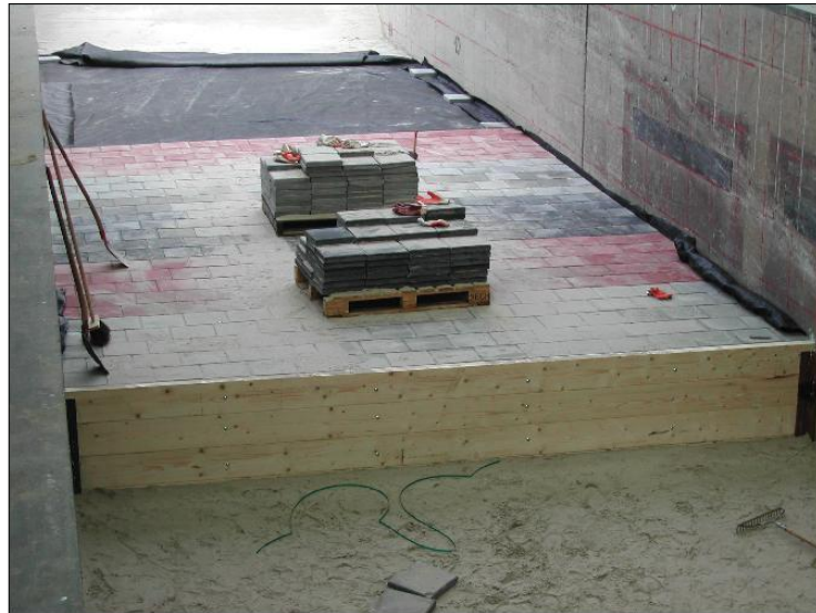
a. Revetment during construction
