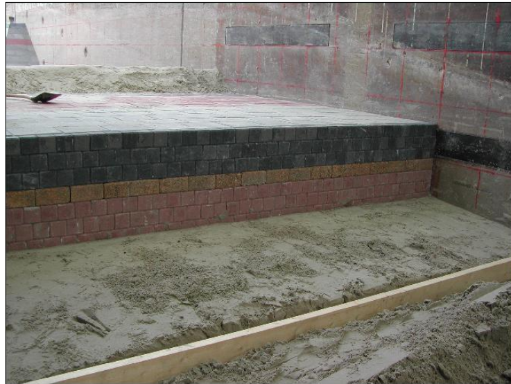
a. Revetment during construction
