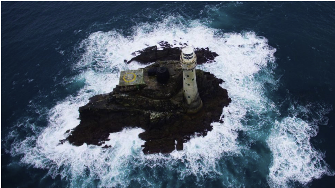
Fig. 1. Drone image of Fastnet lighthouse collected during the field modal test by Mr. James Bassitt (University of Exeter).
