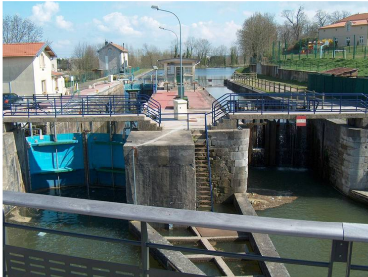
Figure 7.4: right, the lock dating from the origin of the channel (1853) and now abandoned. Left the lock built in 1925 and equipped with composite doors in 2000. (Website: Bord à Bord asbl)
