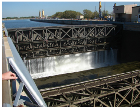
Figure 2.5: Lift gate (USACE [1], 2013, page 7.3)
