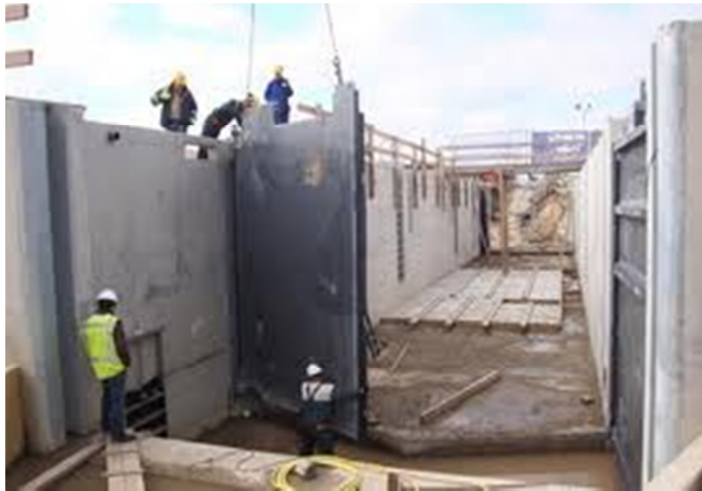
Figure 7.7: Placing of the Erica-Ter Apel gates (FiberCore [1])
