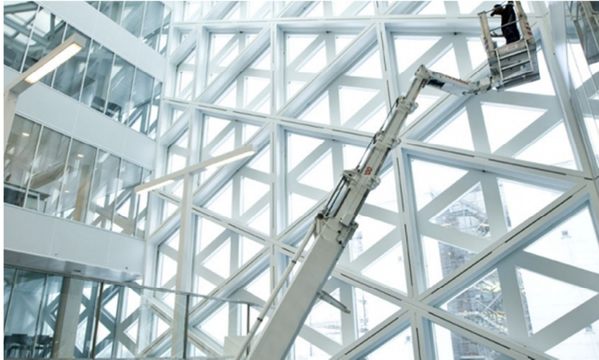
Figure 3.14: Façade Windesheim University as viewed from the inside. (Hollands Composites)
