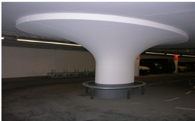
Figure 3.13: Columns in a parking garage under Oosterdokseiland in Amsterdam. ( Nedcam )
