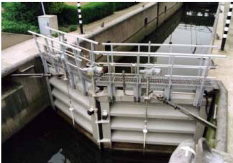
Figure 7.3: Lock gates Spieringsluis. ( Nagtegaal, 2001 )
