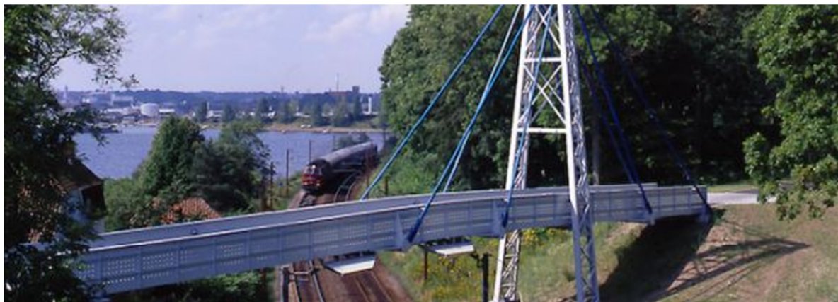
Figure 3.8: Pedestrian and Cyclist Bridge at Kolding in Denmark. (Fiberline [2])
