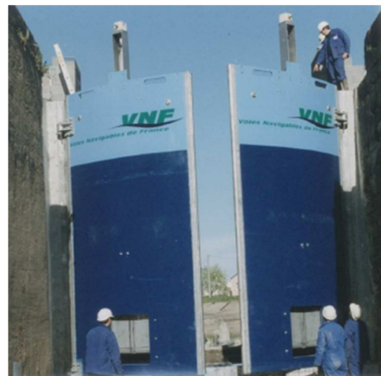
Figure 7.6: Adjustment of composite gates downstream (InCom, 2009, page 18)
