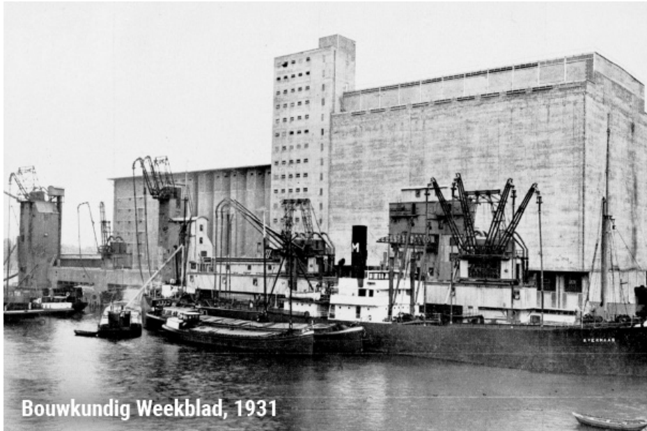
Maassilo: 2nd part after completion
