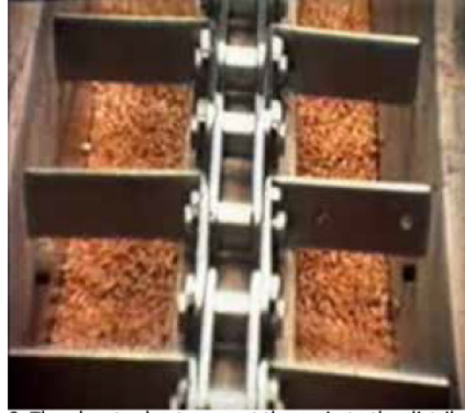
2. The elevator leg transport the grain to the distributing floor
