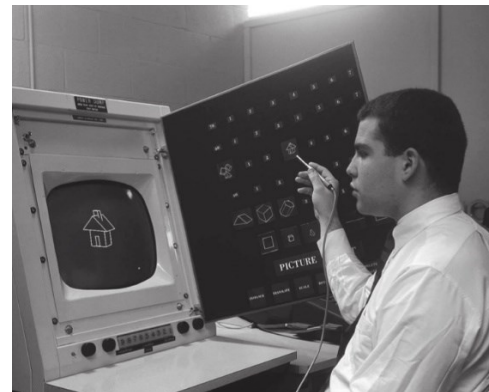
Fig. 10 Lawrence Roberts operating the next-gen Sketchpad-like software with The Lincoln Wand. (MIT Lincoln Laboratory, c. 1966)
