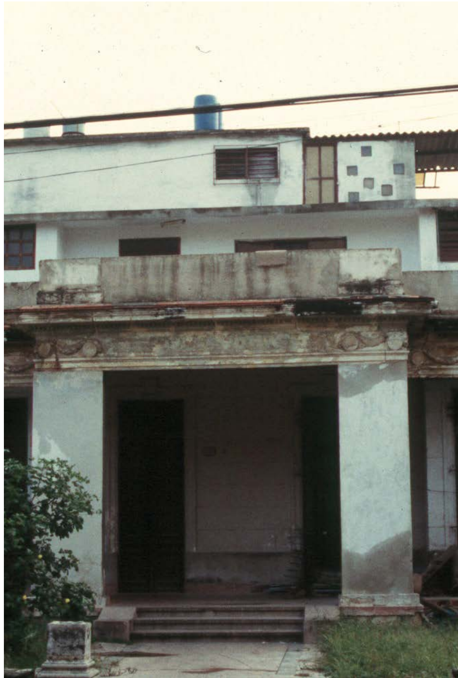
additional construction on the roof
