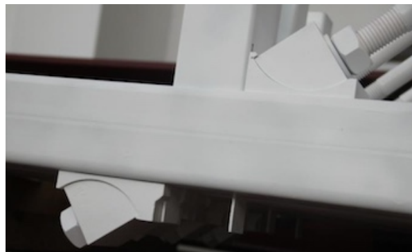
Figure 2.10: Plug & play N type RHS truss connection [41].
