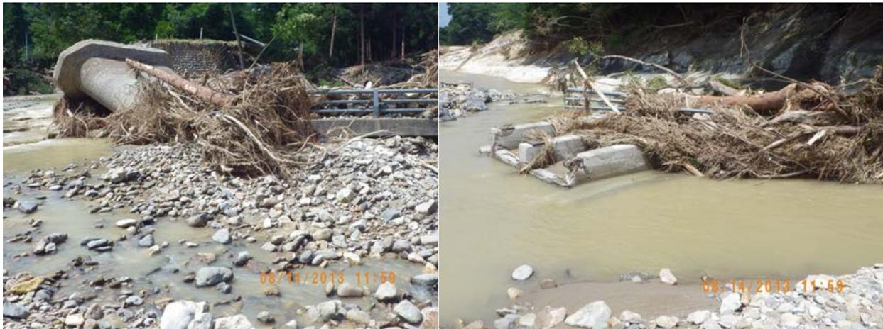
*Figure 1- 4 Collapse of Abashiri River Bridge in Japan (photo by Jeremy Bricker). Indicating the probable role of debris in the collapse process.*
