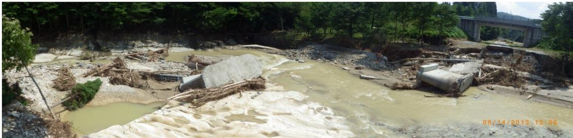
*Figure 1- 3 Collapse of Abashiri River Bridge in Japan (photo by Jeremy Bricker). Indicating that entire pier/girder unit was pushed over by hydrodynamic force.*
