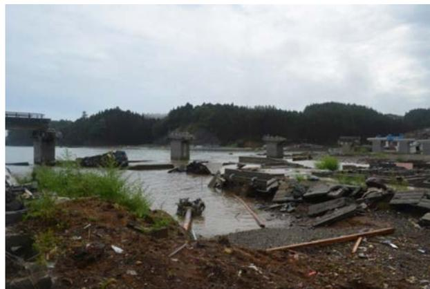
*Figure 2- 11 Utatsu bridge situation after Tohoku Tsunami (2011) [15].*
