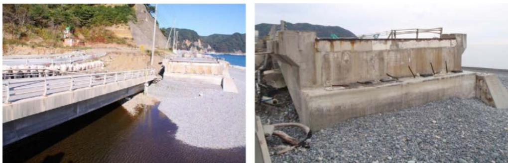
Figure 2- 14 Horizontal movement of bridge deck towards landside during tsunami (left picture). Absence of damage to anchor bars on the seaward side (right picture) [17].
