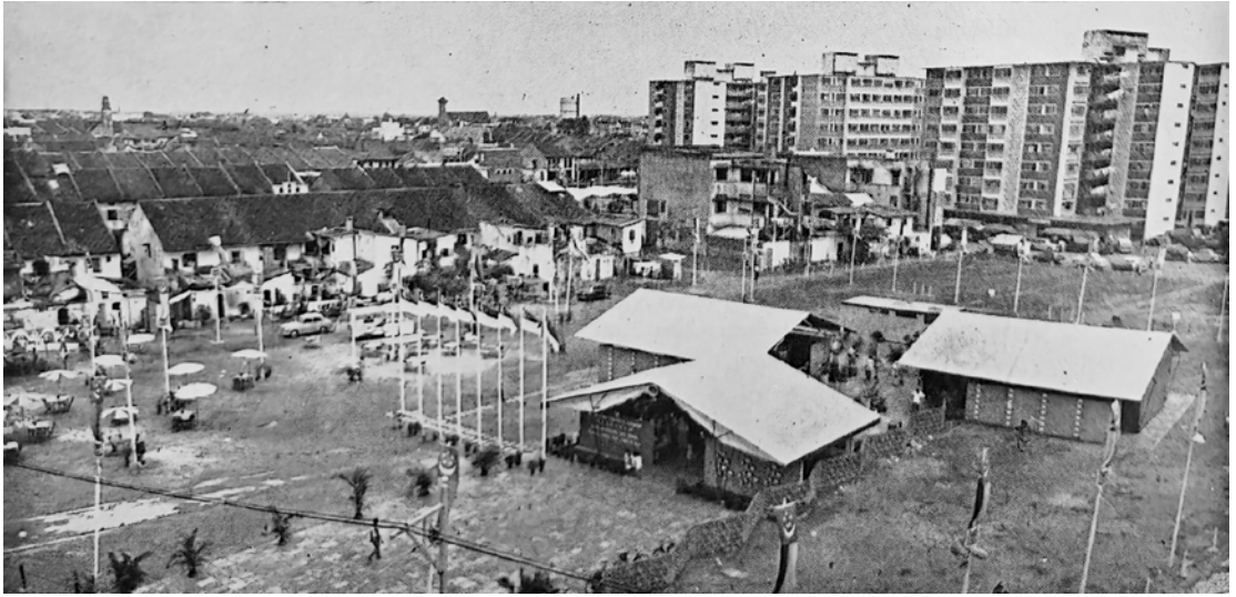
Fig. 10 Photograph of HDB Low-Cost Housing Exhibition on the Selegie House site, 1960. Source: Rumah Journal of the Singapore Institute of Architects (1961) / National Library Board Singapore.
