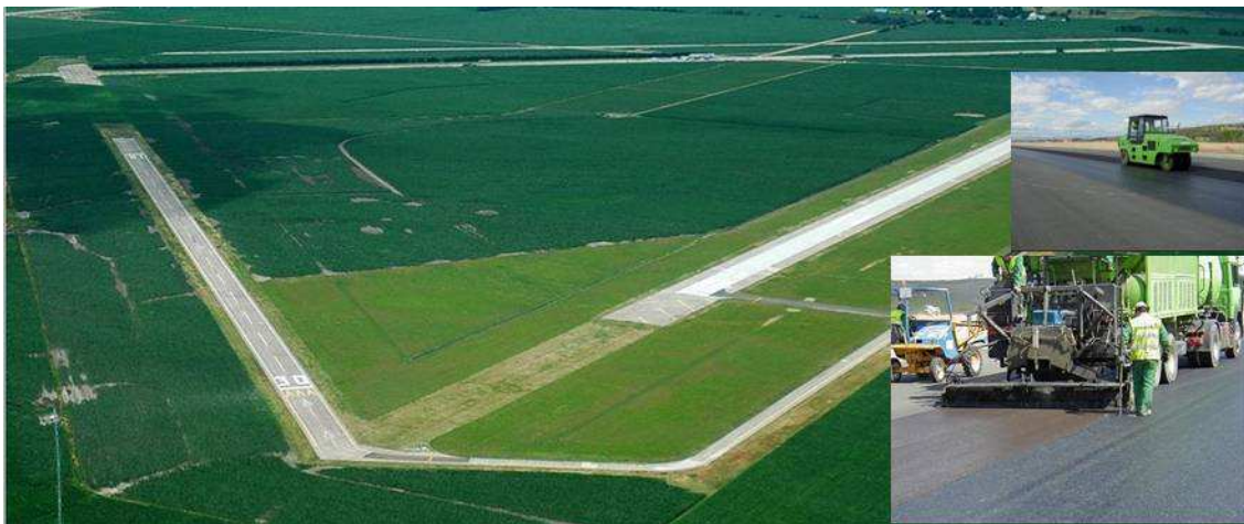
Figure 1 Construction of antiskid layer on the airfield
