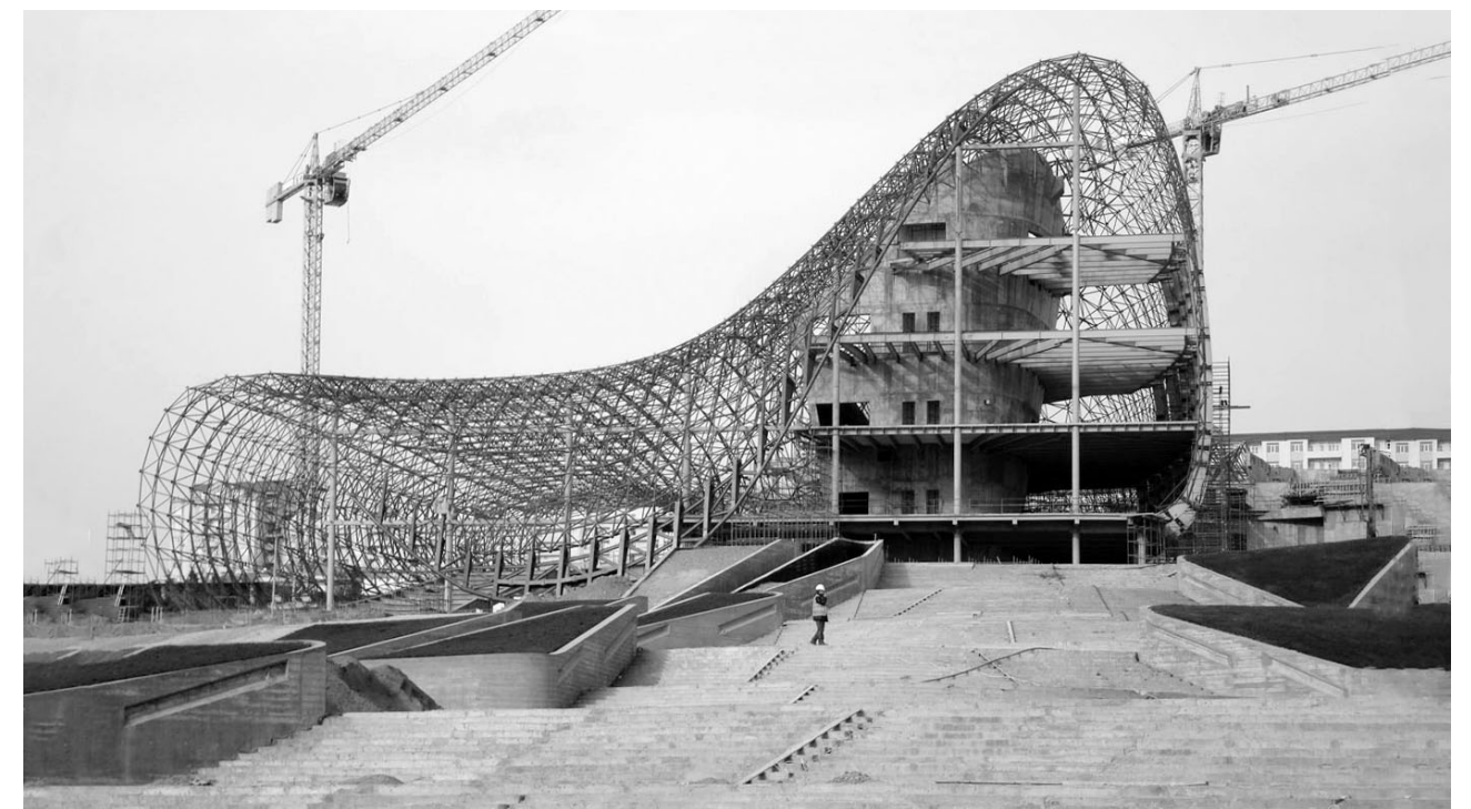
Figure 6. Zaha Hadid's Heydar Aliyev Cultural Centre construction. (Zaha Hadid Architects, 2011).
