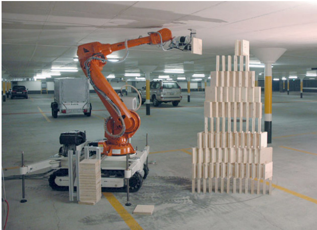
Figure 19. In Situ Robotic Fabrication in which the robot recognizes its own position, the surroundings, and its components with regard to the material tolerances. (Gramazio Kohler Research, ETH Zurich, 2012).
