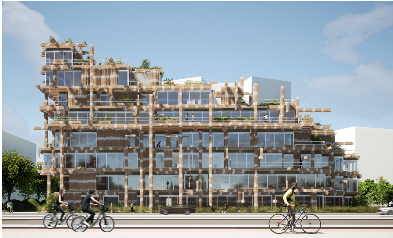
Figure 79. Facade viewing the Laan op Zuid Avenue (by author, 2023).
