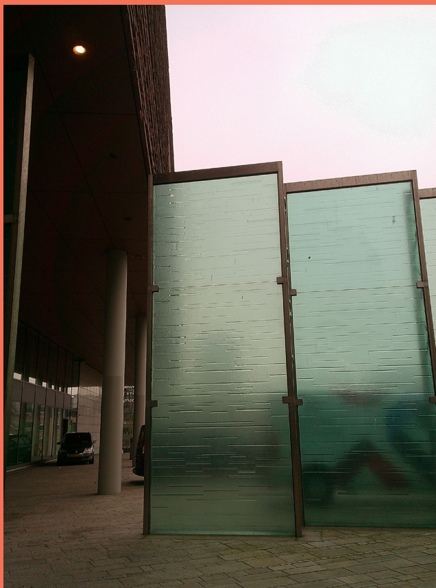
Glass plates keeping out the noise and sight of the traffic behind
