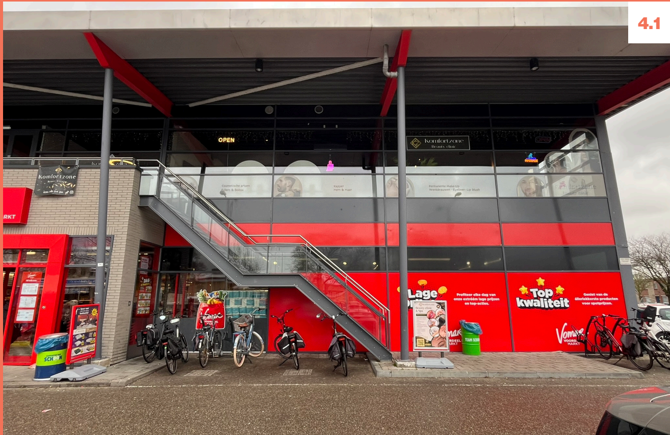
Stairs keep the bike parking semi-dry
