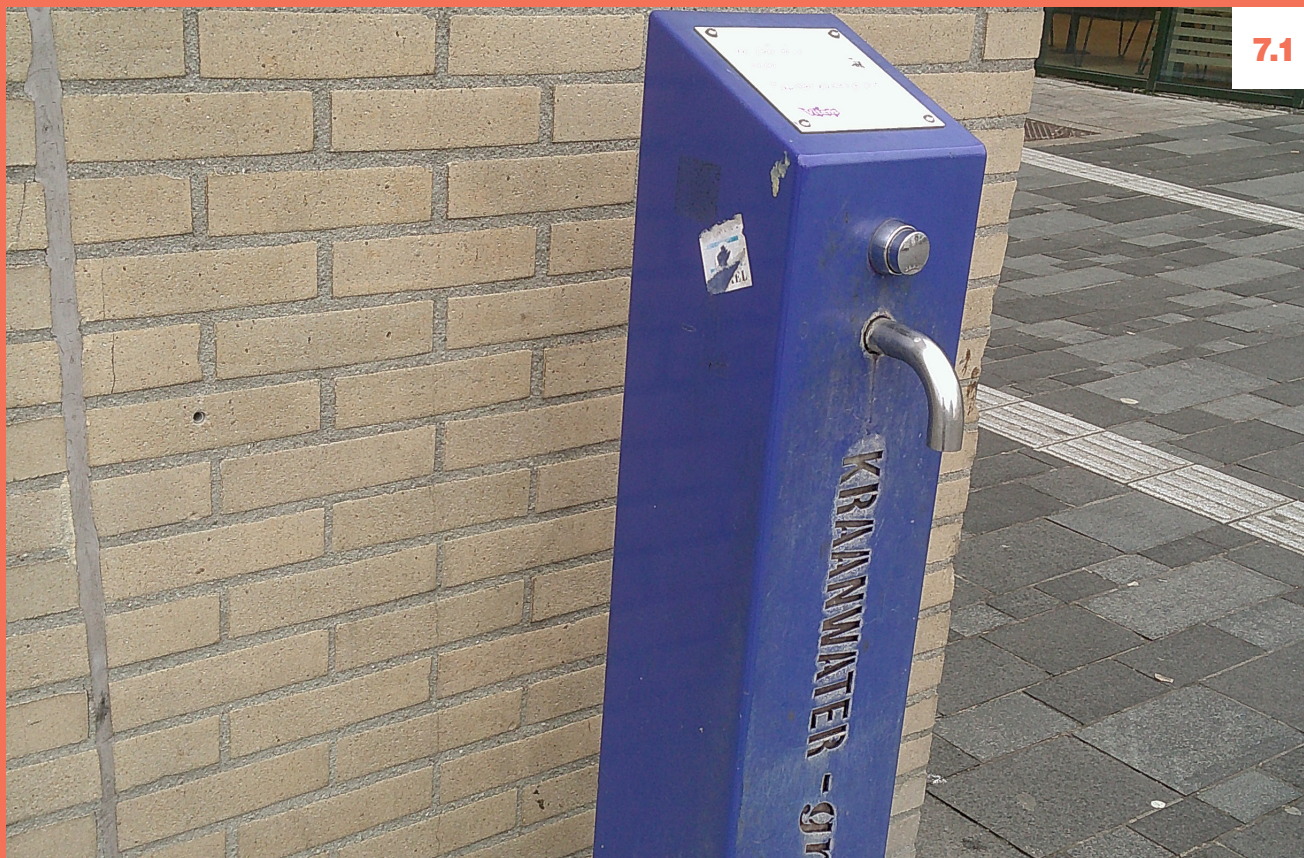
Tapwater station at the marketsquare "Kraanwater - graag"
