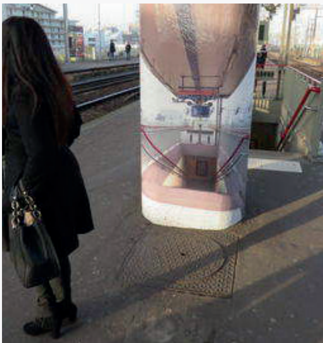
► Fig. 17 - A photosticker of the stairs on a pillar, to increase the visibility of the exit.
