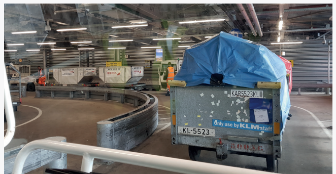
► Fig. 21 - Blockade in the baggage basement. On the left there are dollies with loading units, in front are baggage carts.
