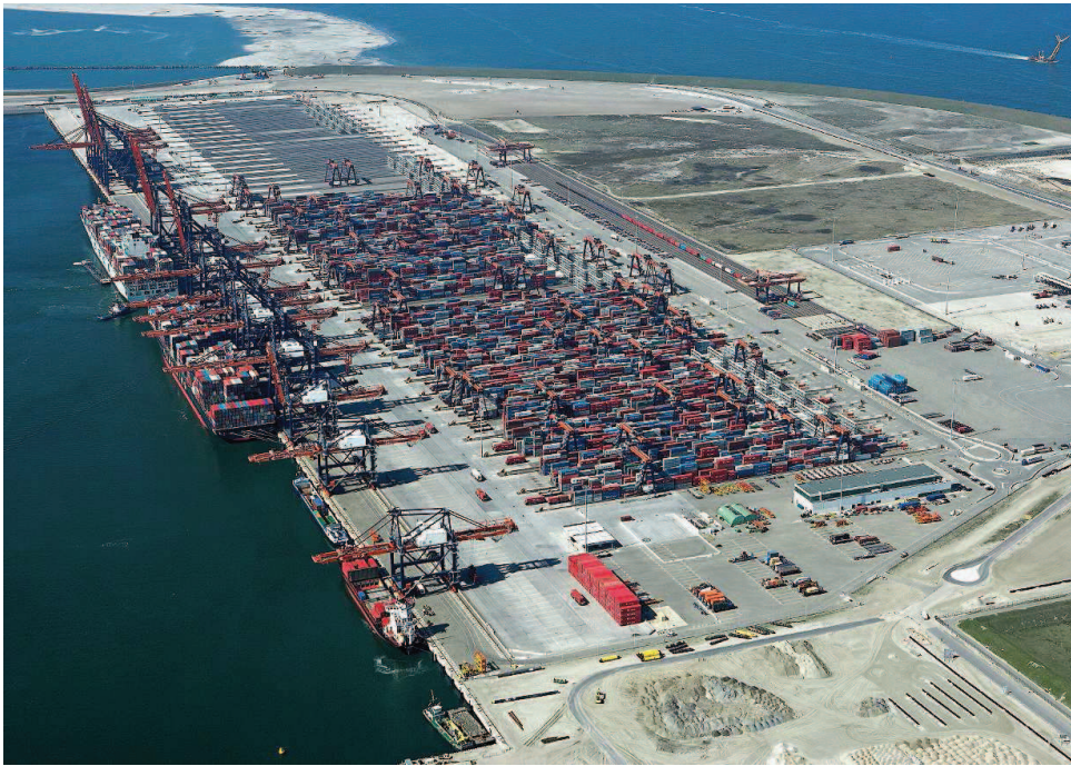
Figure 1.2: The Euromax container terminal (Courtesy of ECT).
