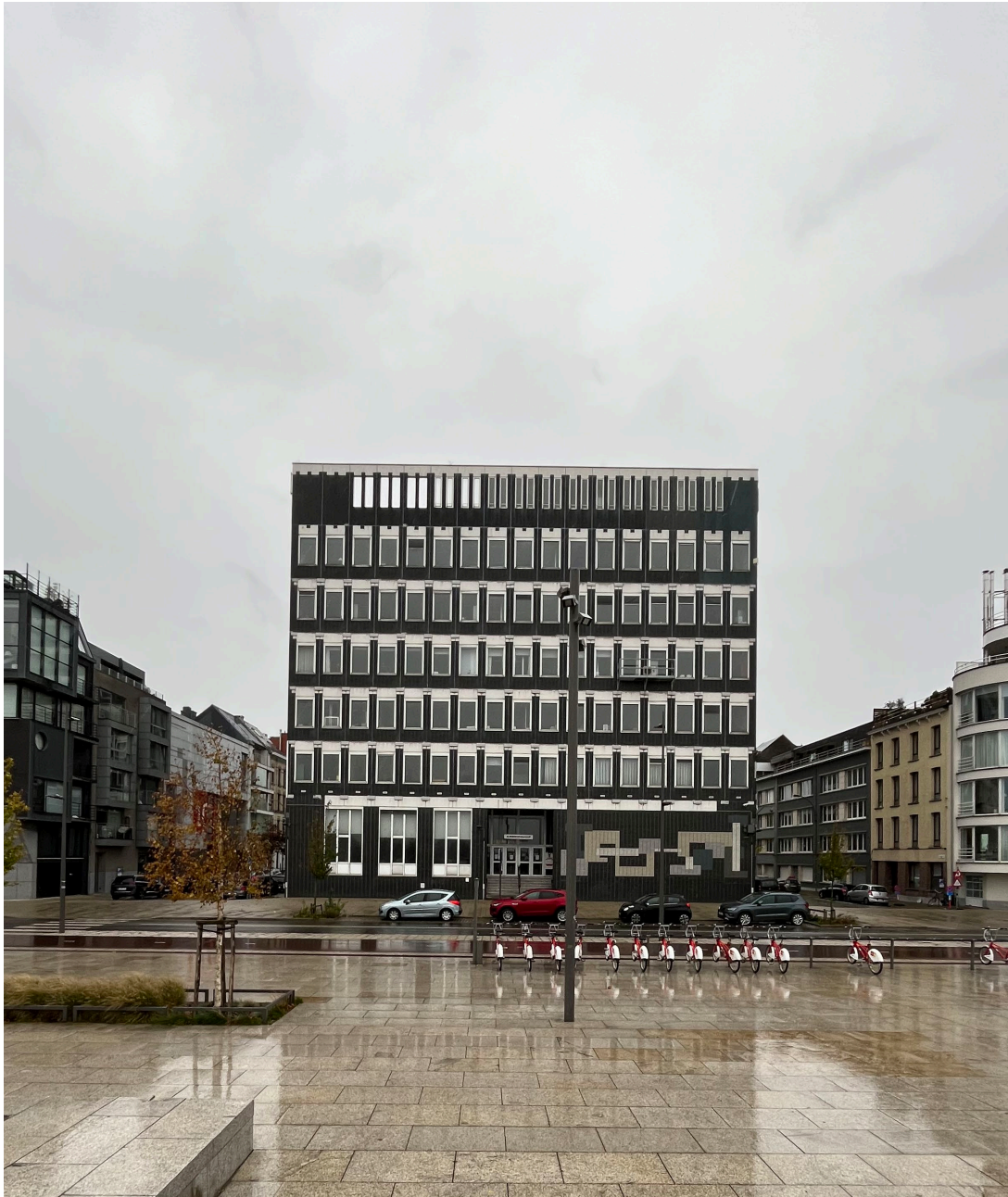
existing building in its context
