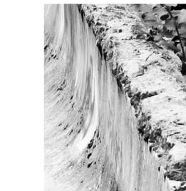
The insulation material is still visible on some places of the bobsleigh track, although crumbled.
