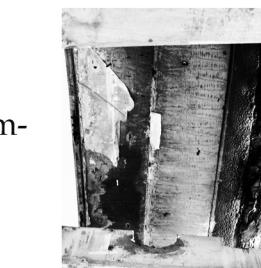
The bottom of the track is covered in a reddish substance: rust. You can also still see the holes through which the ammonia used to be pumped.
