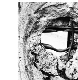
These holes, caused by shelling during the war, show the structure of the track: reinforced concrete.
