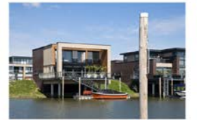
Houses are elevated to accommodate high water
