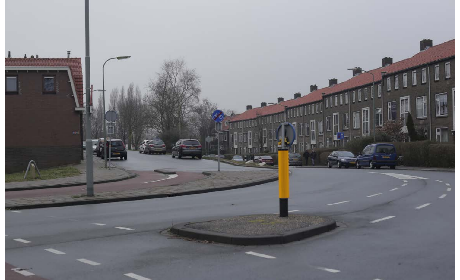
Fig.14 Residential townhouses along the Zuidendijk with different levels as the dike is no longer part of the outer dike. Source: Author's photograph
