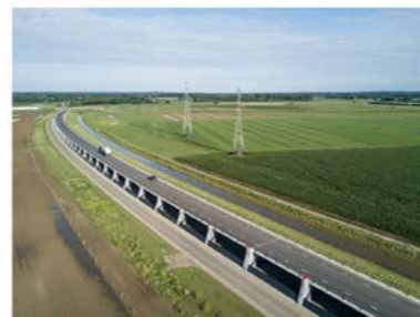
New bridge as accessway when the bypass is used.
