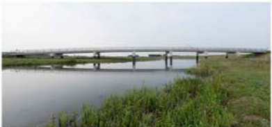
Bridges are constructed to join the separated polders
