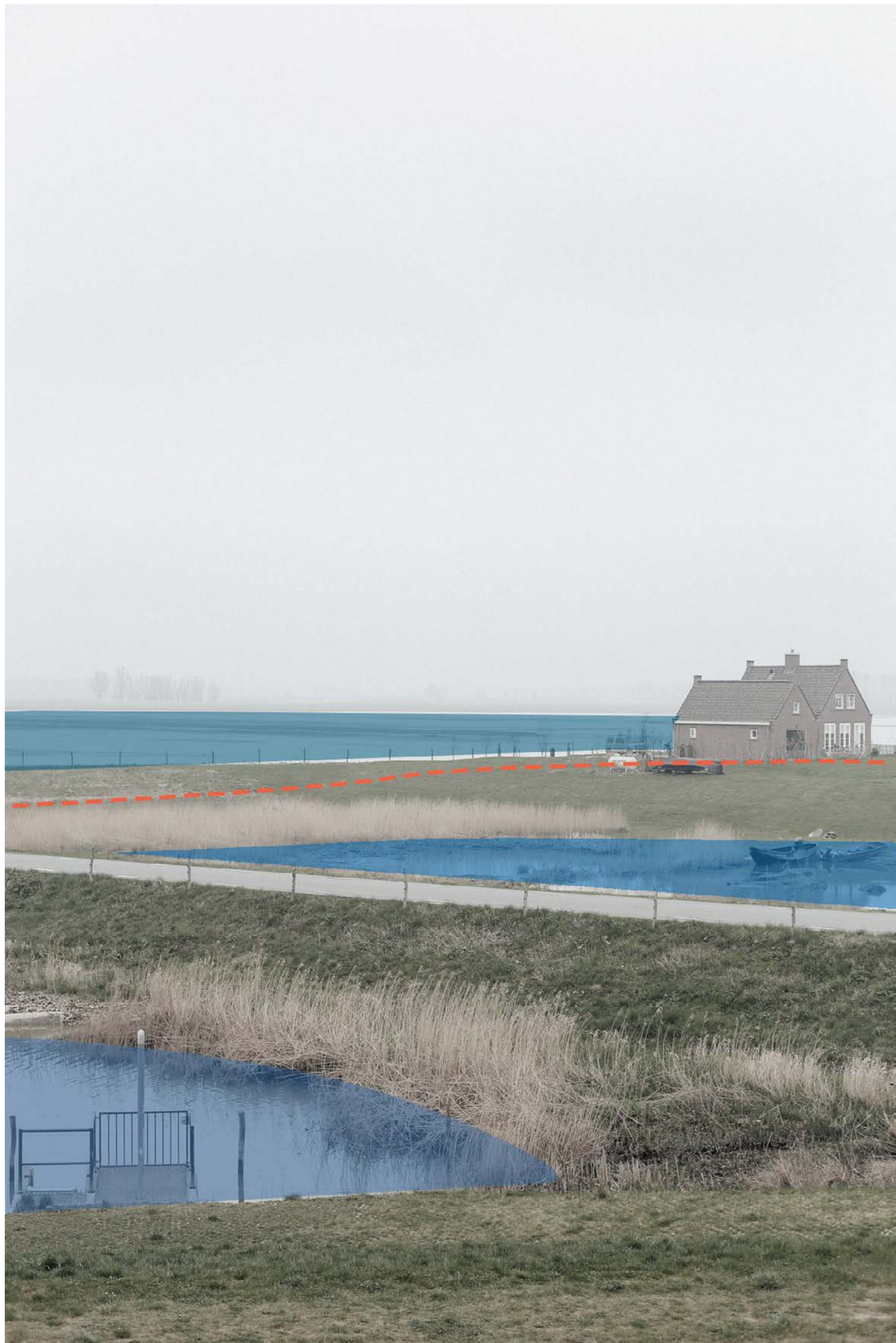
Fig. 29 Farm house on top of a new mound as part of depoldering Noordwaard project. 3 different water level can be seen in this picture; polder level, intermediate level, and tidal river level. This project creates room for water fluctuation whilst restoring the ecological qualities of the landscape.
