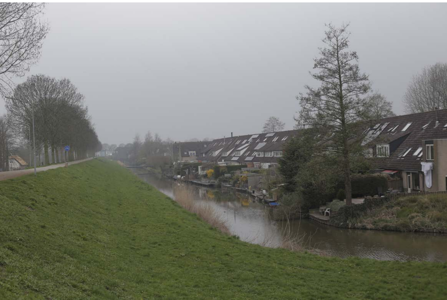
Fig. 15 Striking height difference of protective dike and residential areas around it. Source: Author's photograph
