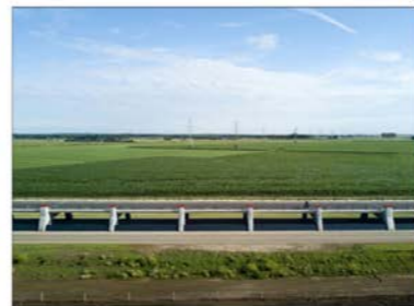
Beneath the bridge is the inlet that can be manually operated to allow flood water to come in.
