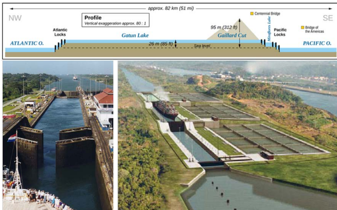
Figure 1.5: The Panama Canal. Top: longitudinal profile; bottom left: the oldest Gatún locks (Atlantic lock system); bottom right: the newest Cocoli locks (Pacific lock system) (source top panel: Panama Canal Map EN by Thomas Rmer is licenced under CC BY-SA 2.0; source bottom panels: Panama Canal Gatun Locks opening by Stan Shebs is licenced under CC BY-SA 3.0 and ACP conceptual view of the Third Set of Locks 02 by Autoridad del Canal de Panama is licenced under CC0 1.0).
