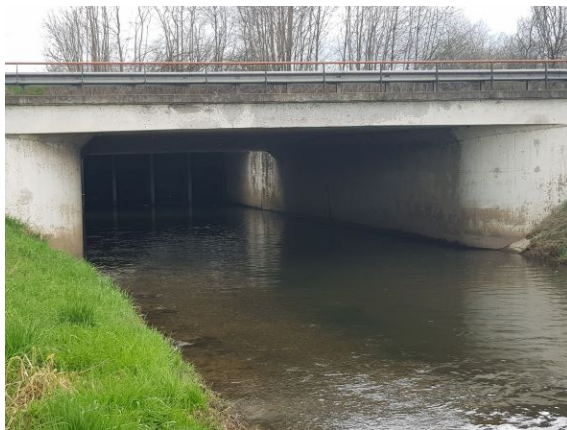
Figure A.8: Inlet of the Tungalroyse beek inverted siphon
