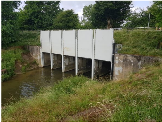
Figure A.4: Inlet of the Geul inverted siphon
