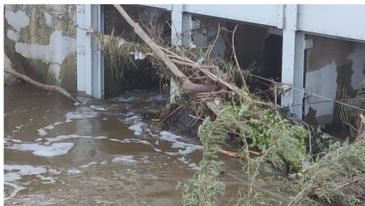
Figure 1.2: Debris at the Geul inverted siphon (2) (Deltares, 2022)
