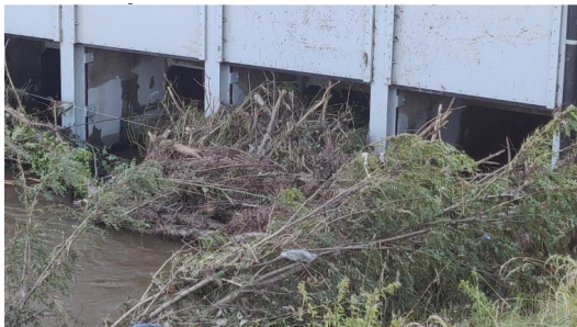
Figure 1.1: Debris at the Geul inverted siphon (1) (Deltares, 2022)
