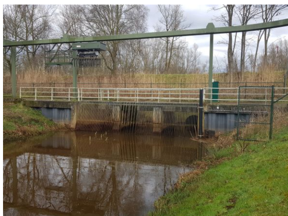
Figure A.1: Inlet of the Tungalroyse beek inverted siphon
