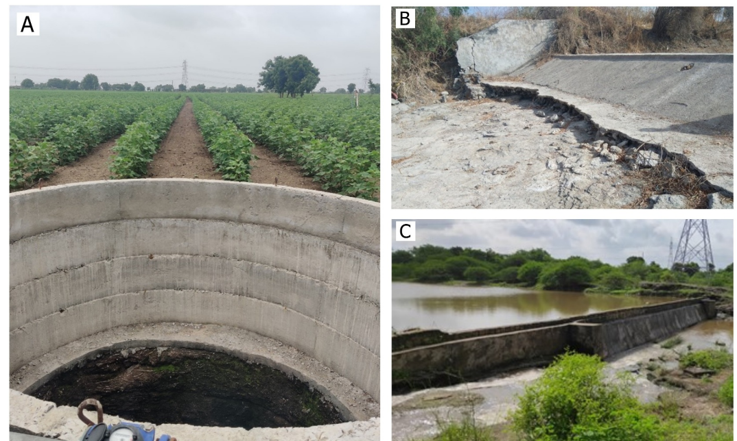
Figure 2. (a) Open dugwell commonly used for irrigation in the study area; (b) and (c) check dam in the area in dry and wet season, respectively (images taken from downstream side).
