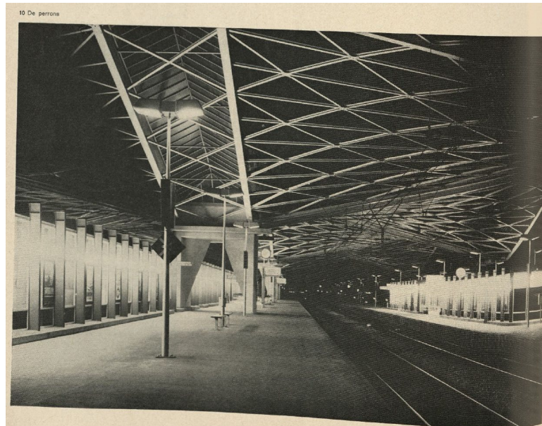
Photo of platform in the Station Tilburg, 1966 34
