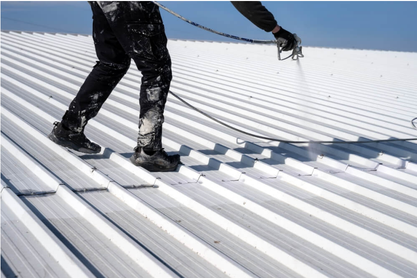
Aluminium roof with acrylic coating has a high UV reflectivity. From "What Is the Best Coating for Metal Roofs?" (Perfect Exteriors, 2024)
