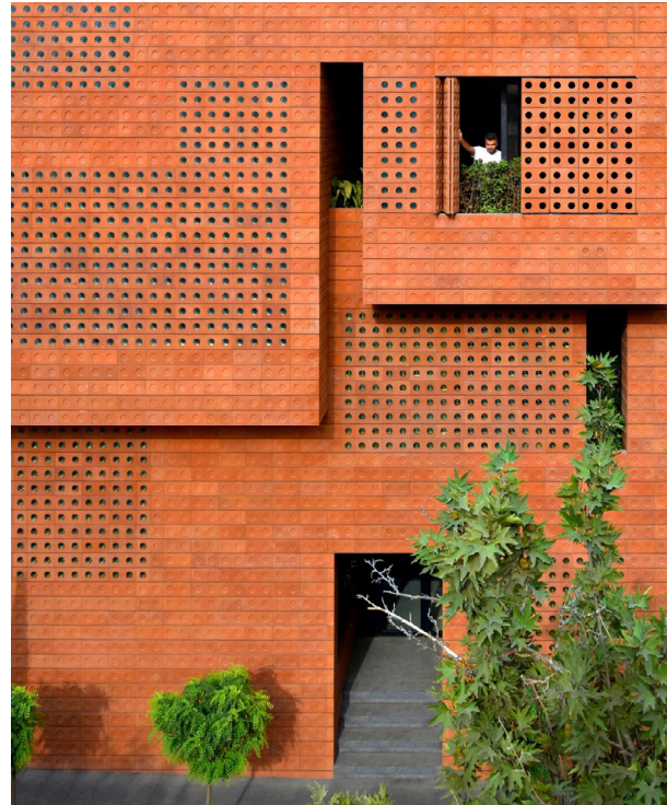
Semi-transparent brick facade. From "Hooba Design Group wraps Tehran office in glass-punctuated bricks" (dezeen, 2020).
