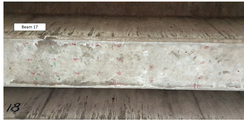
Figure 6.4: Template for marking test locations
