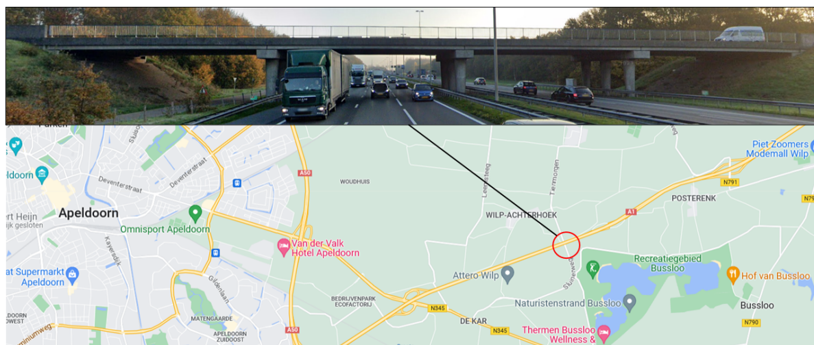
Figure 5.1: Sluinerweg viaduct (KW03), A1
