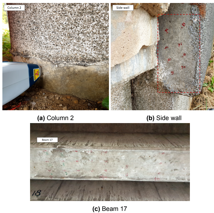
Figure 5.6: Measured concrete structural members and measurement points
