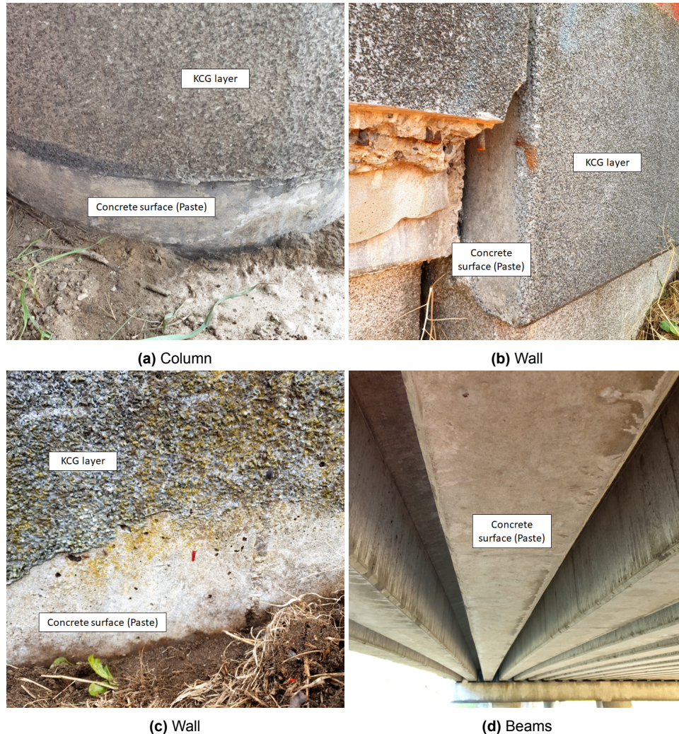
Figure 5.4: Identification of concrete surfaces without KCG layer for testing with hXRF
