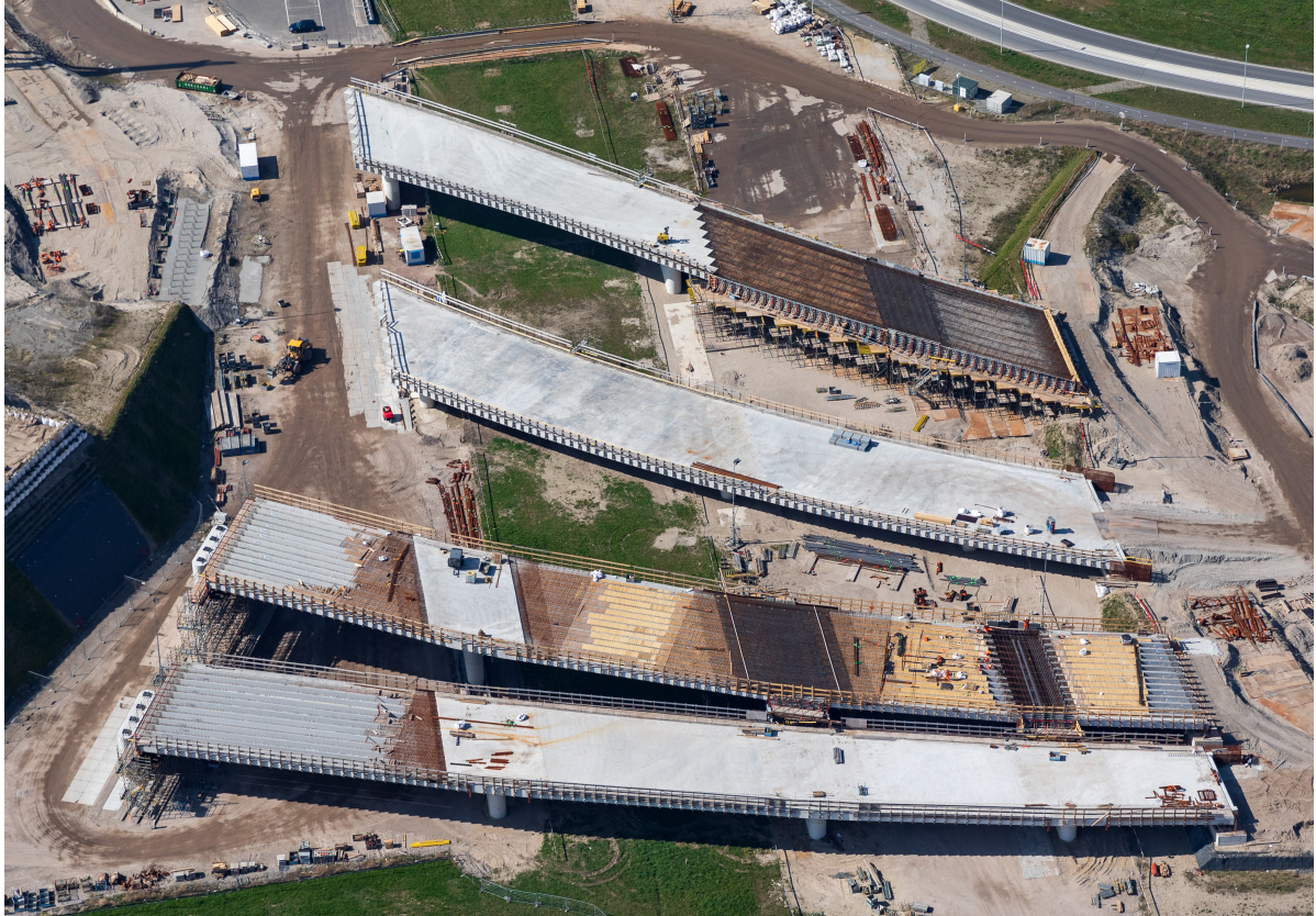
Figure 2.8: Top view of Blankenburg viaducts under construction (March 2021)
