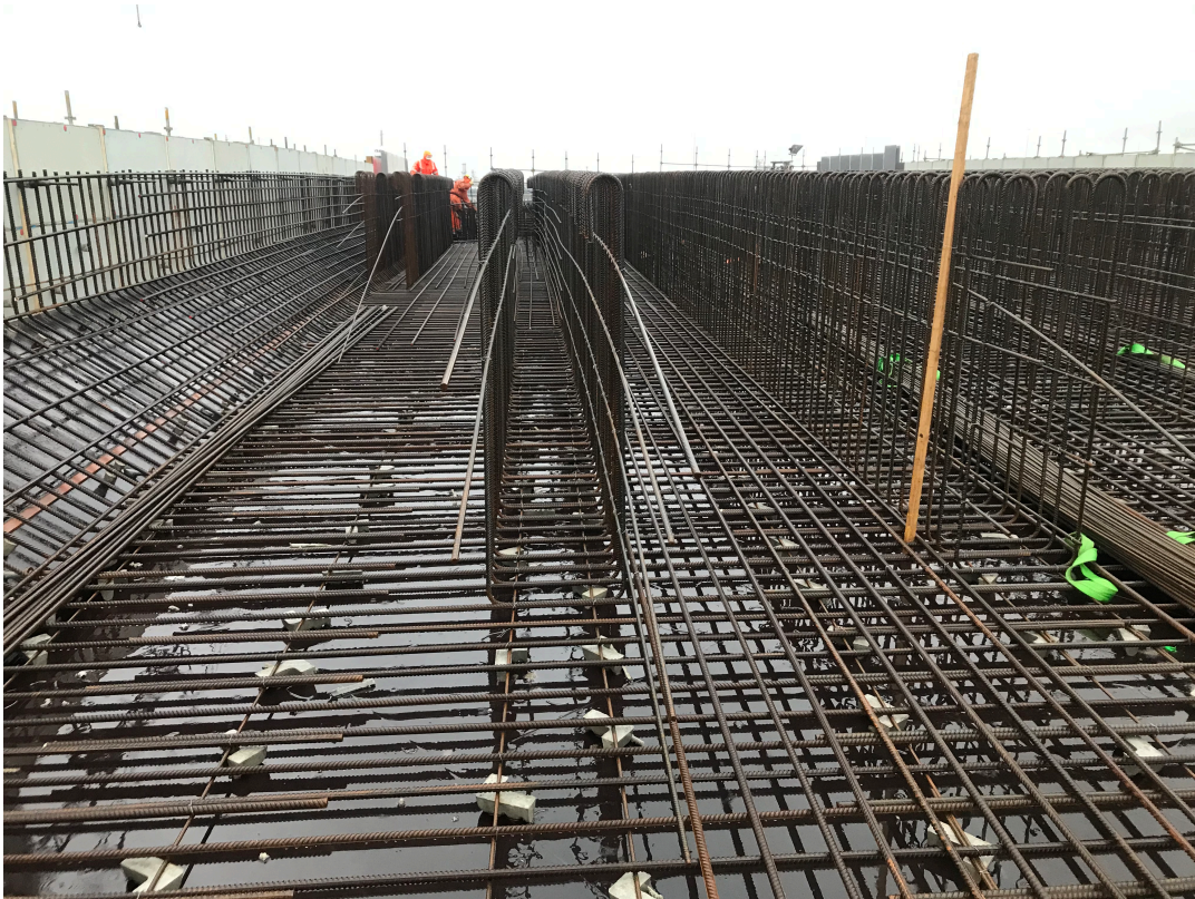
Figure 2.5: Transverse, longitudinal and shear reinforcement
