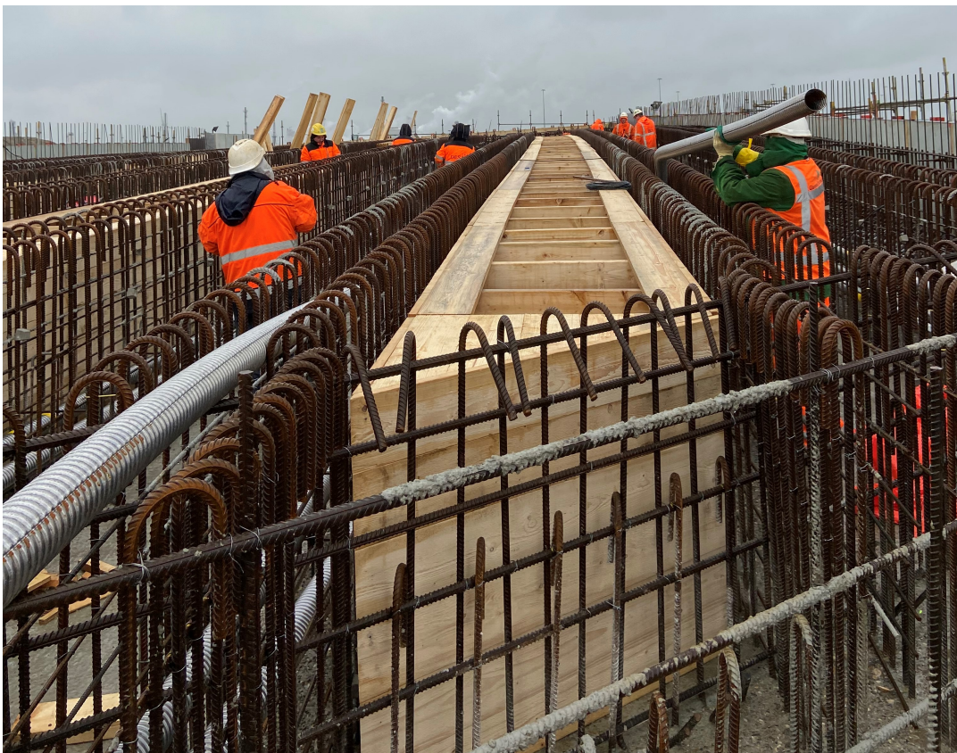
Figure 2.6: Formwork for the voids and installation of casing pipes for pre-stressing
