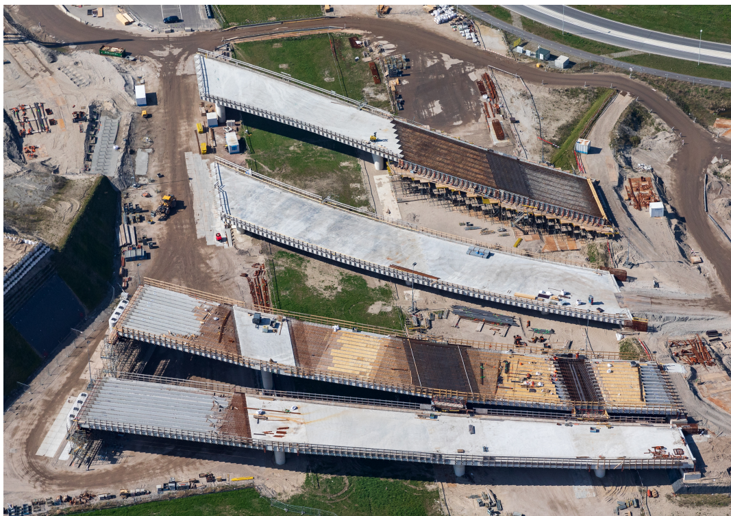
Figure 1.3: Top view bridge decks under construction (March 2021)
