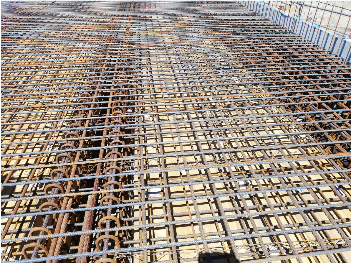
Figure 2.7: Reinforcement top plate, hairpins and formwork of the voids
