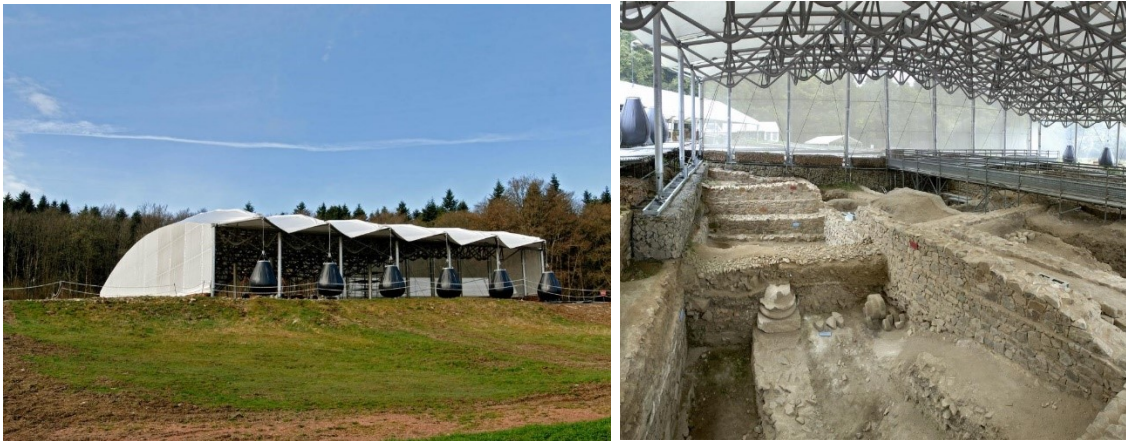
Figure 1,2. Archaeological shelter at Bibracte, France. Exterior view with the black ballasts. Interior view of the excavation site and the scaffolding corridor for the visitors.
