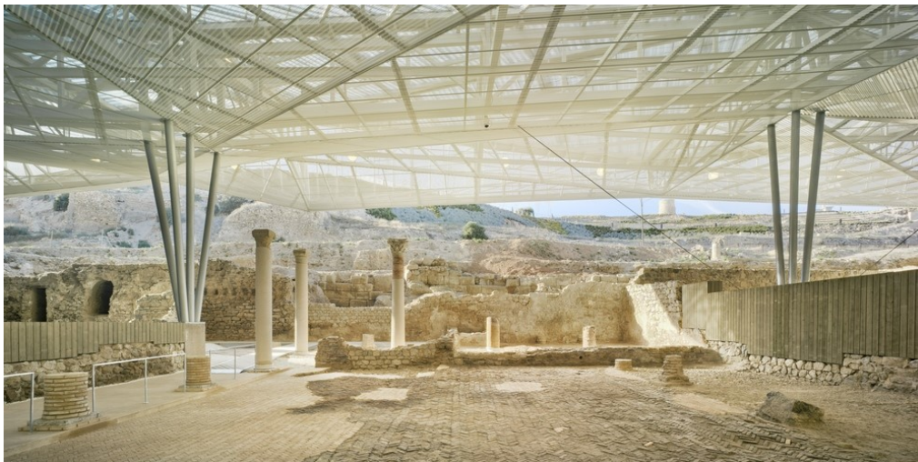
Figure 11. Inner view of the canopy from the level of the visitor over the archaeological remains.
