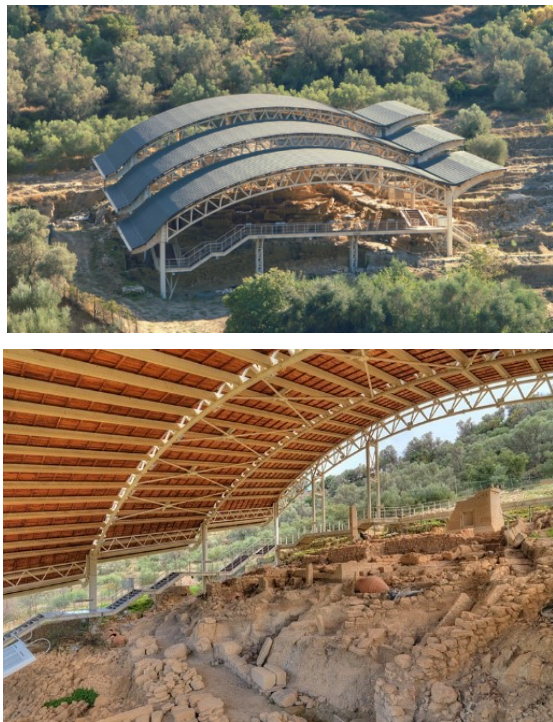
Figure 12,13. The Eleutherna shelter. Overall view and view below the roof.
