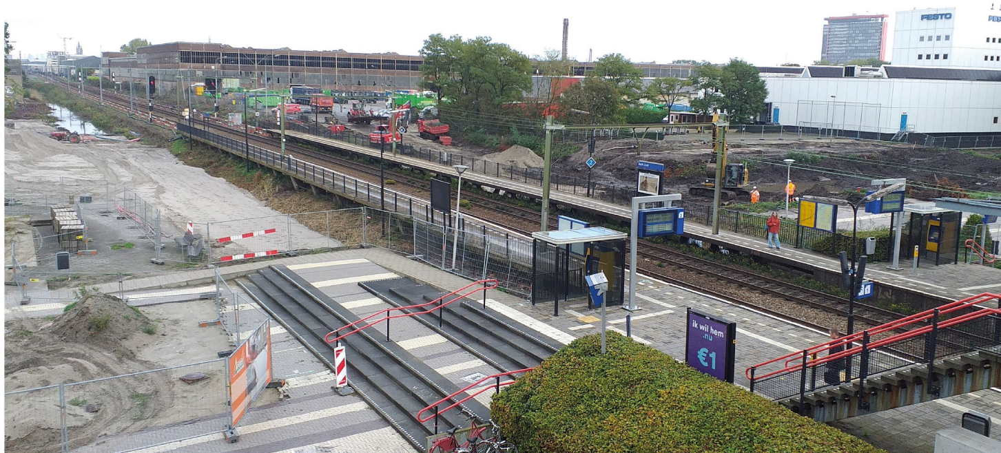
Building site for the new tunnel of Delft Campus station source: author (yesterday)
