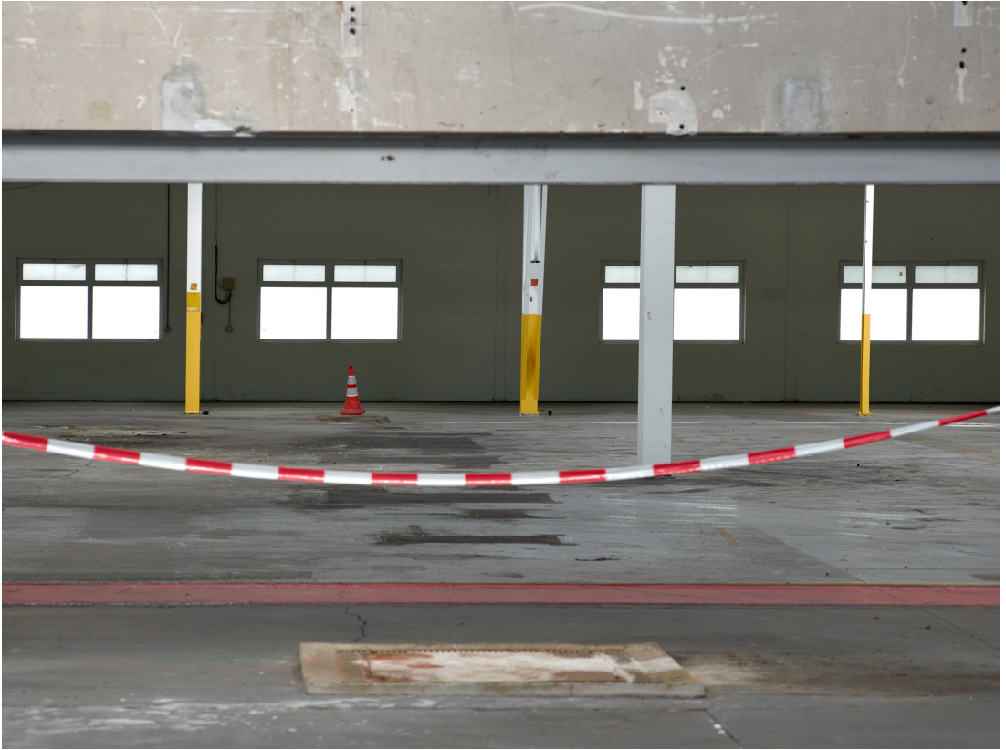
photos provided by Blikfabriek
