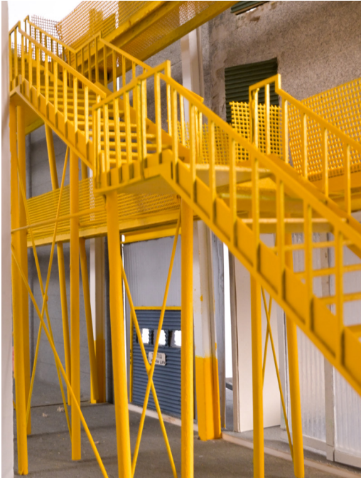
2028, covered back street with staircase
