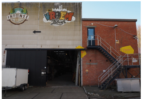
2024, service access back
