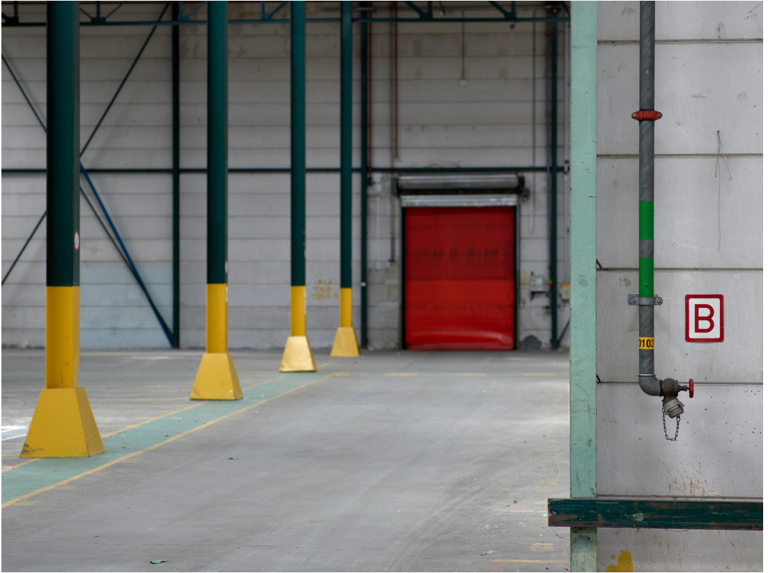
photos provided by Blikfabriek
