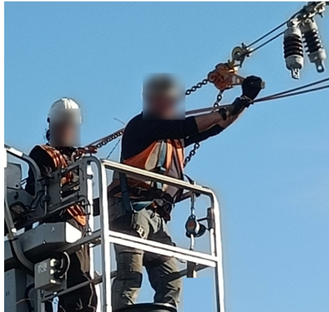
Figure 5.14: The process of tensioning the contact wire with the chain hoist. The worker connects the end of the chain hoist to the isolators and to the contact wire. By pulling the chain hoist the wire is brought to the desired mechanical tension.
