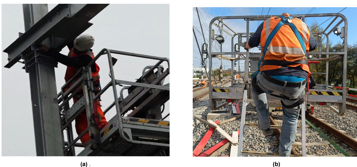
Figure 5.22: a) The worker secures the clamp on the top bar. The boom lift is not moved around the pole while doing this. b) A worker getting into the working platform on a boom lift.
