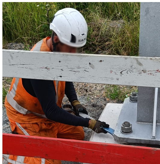
Figure 5.6: The process of securing the pole on the foundation. The bolts are secured manually with a wrench.
