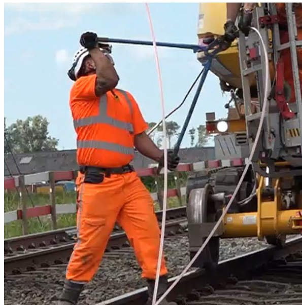
Figure 5.3: A worker cutting a contact wire with a bolt cutter.
