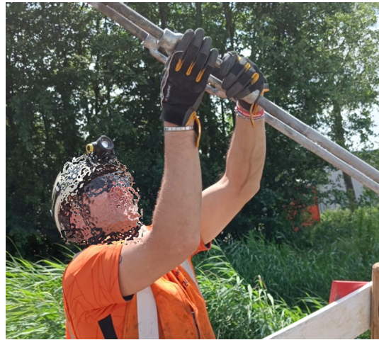
Figure 5.7: The process of manually tensioning a pulling brace.
