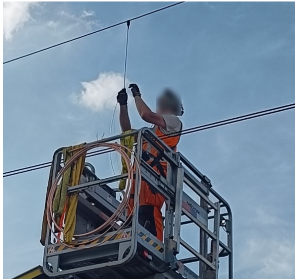
Figure 5.16: The process of installing drop wires between the messenger wire and the contact wire. The drop wire is manually secured to the messenger wire and contact wire.
