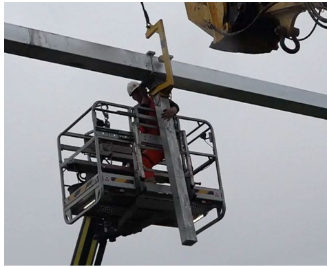
Figure 5.10: The process of installing a drop post onto the top bar. The excavator lifts the drop post and the workers coordinates the drop bar to the right position and secures it to the top bar with a power tool.
