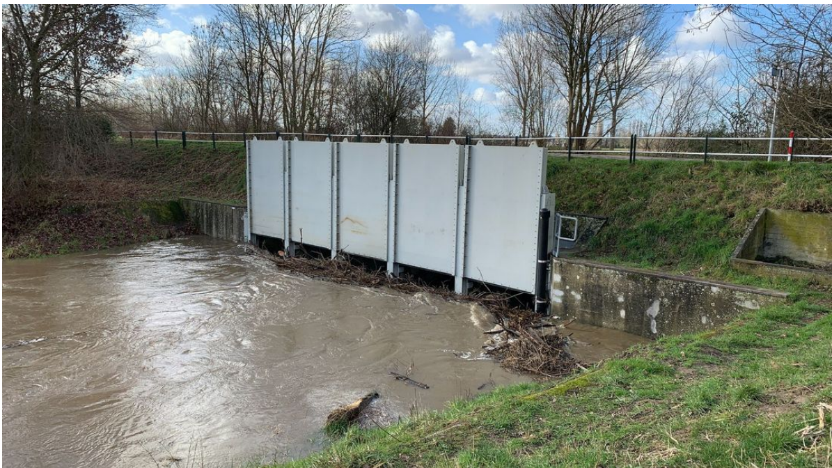
Figure 1.1: The inverted siphon at Bunde under the Juliana Canal during high water, Abeling [2022]
