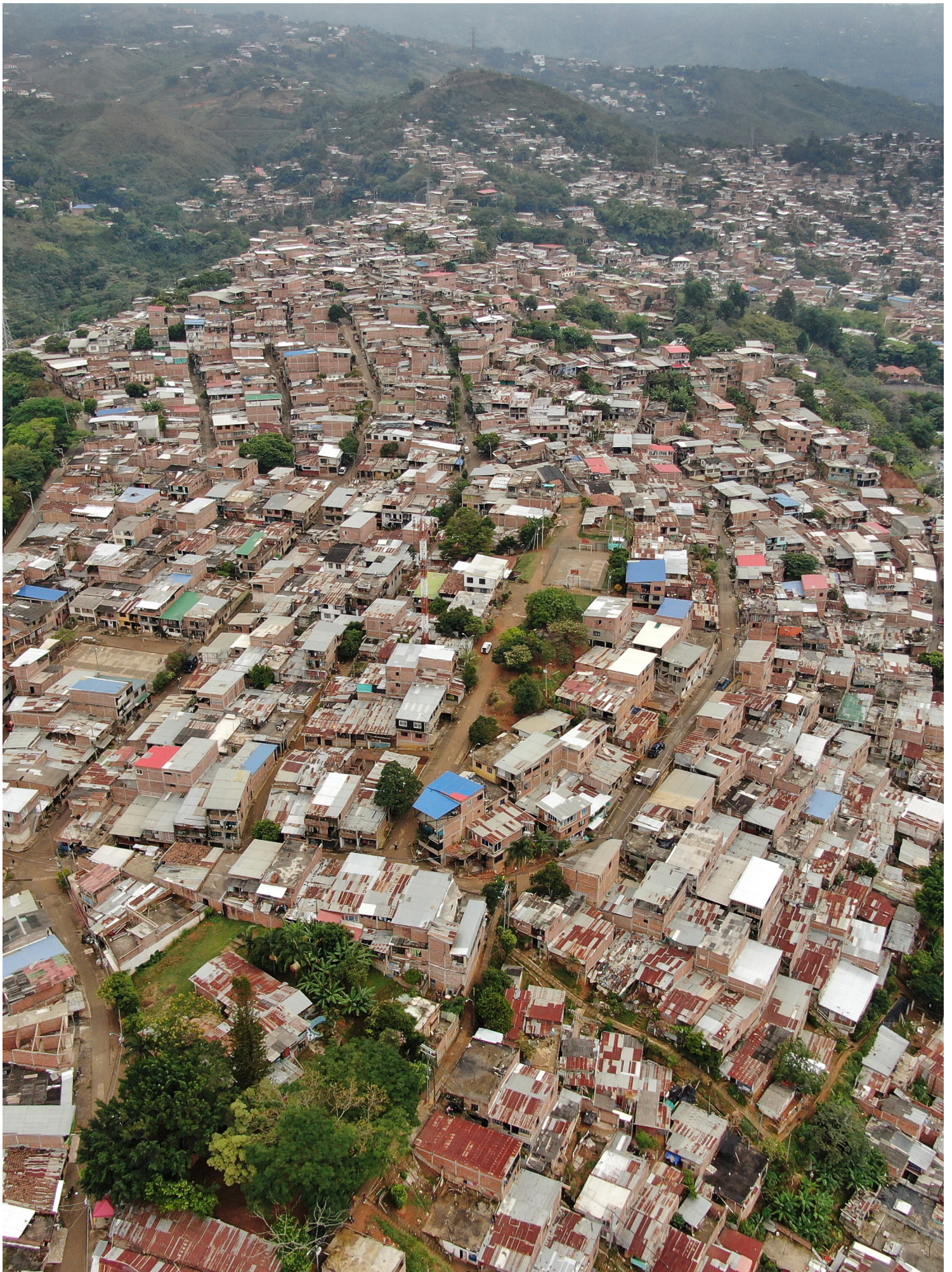
Fig. 51 Aerial image of Comuna 13, located in the western area of Cali. Picture by Monoceja.
