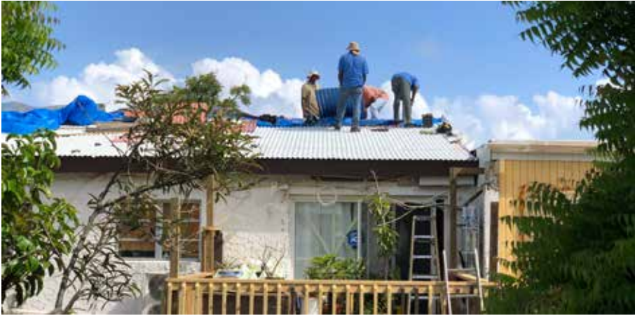
Figure 106: A group of men replacing the tarpaulin on the roof with corrugated zinc plates.
