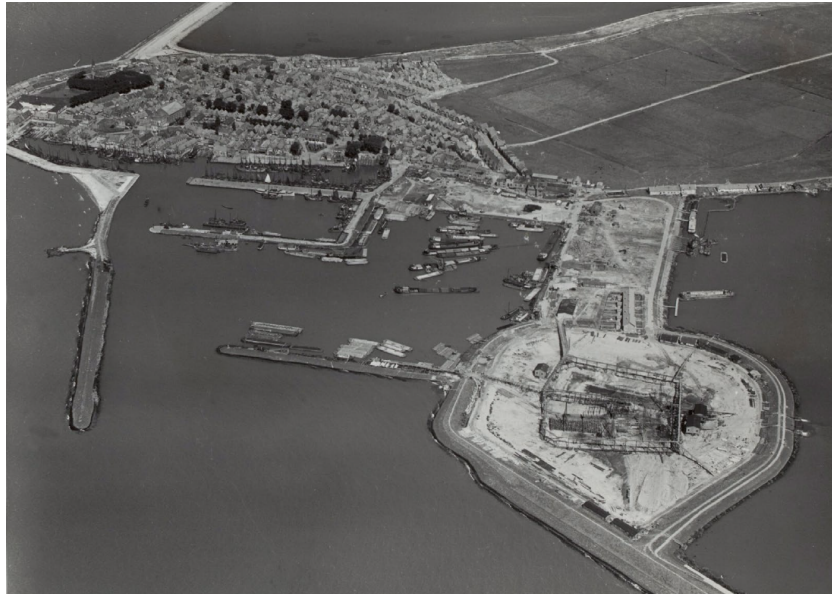
Figure 3.2: The island of Urk, including the two dikes connecting it to the mainland in the north (top left) and east (bottom right), along with a work island and a lock under construction (Post & Post, 2018).
