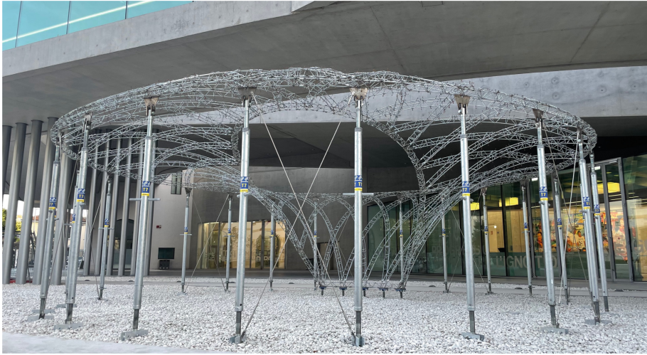
Fig. 10. Demonstrator in the construction stage of the completed gridshell made of bending-active splines.
