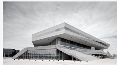
Urban Mediaspace By SHL architects, designed as a big covered public space, which offers the flexibility needed for the new generation of libraries. The program is 30 000 m 2 and contains a theatre, library, media, offices, restaurants and parking spaces.
