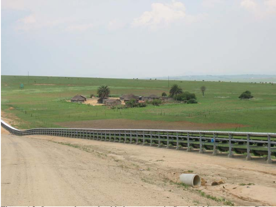
Figure 6.3: Large scale overland belt conveyor in South Africa (courtesy Conveyor Experts B.V.).
