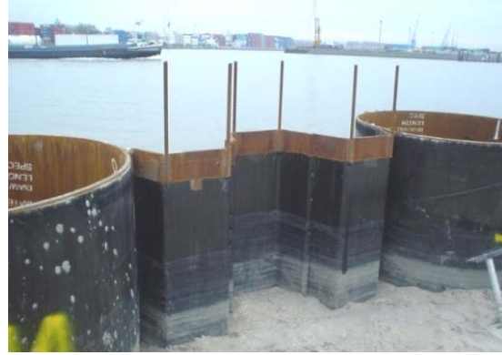
Fig. 1: Schematic and photo of a combined wall of tubes and infill sheeting, also called CombiWall; the infill sheeting is connected to the tubes with welded slots
