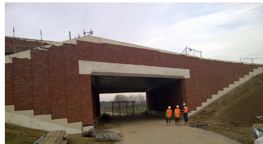
Fig. 4: Brickwork at the Oosterhoutsedijk
