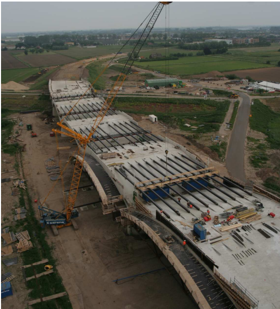
Fig. 6: Prestressed beams between the crests
