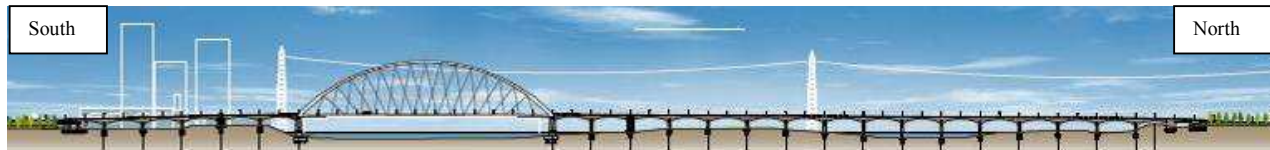
Fig. 2: View of the bridge
