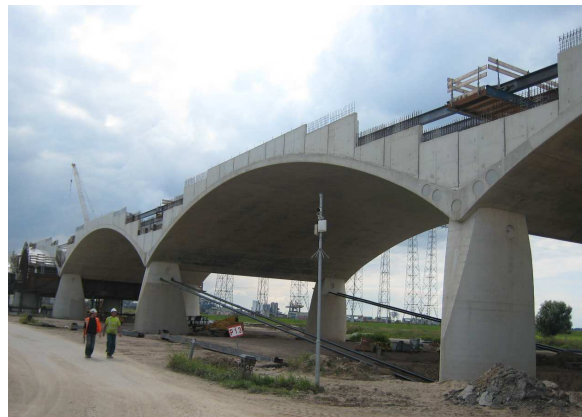
Fig. 7: Prestressed tendons at PN7-PN8
