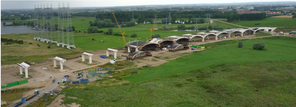
Fig. 5: Columns, hammerheads and falsework
