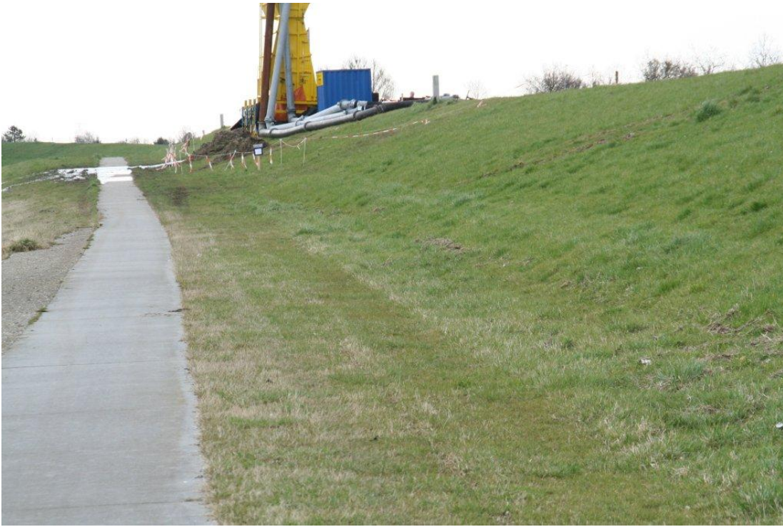
Figure 2.8. Kattendijke - Eastern Scheldt. Seaward side, protected down slope 1:3.5, berm 1:20 with foot or cycle path and partly grassed slope, upper grassed slope 1:3.0.
