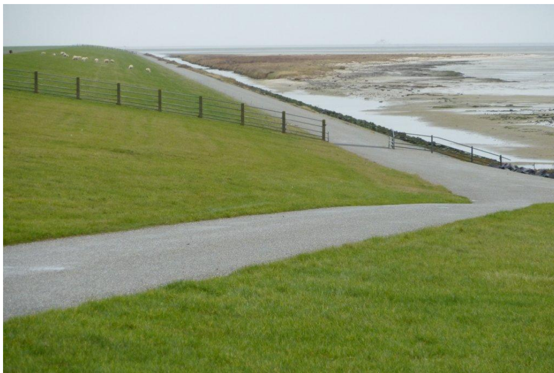
Figure 2.16. Dike at Ameland. Protected slope below 2 m +NAP, then a cycling path as berm. Upper slope about 1:5. Design water level 4.5 m +NAP; design wave height 1.6 m.
