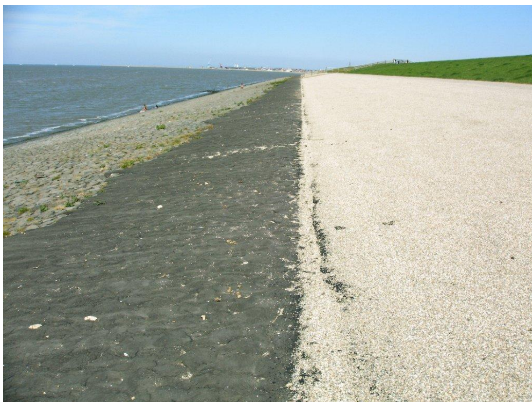
Figure 2.10. Dike between Harlingen and Afsluitdijk. Design water level 5.0 m +NAP; design wave height 2.2 m.
