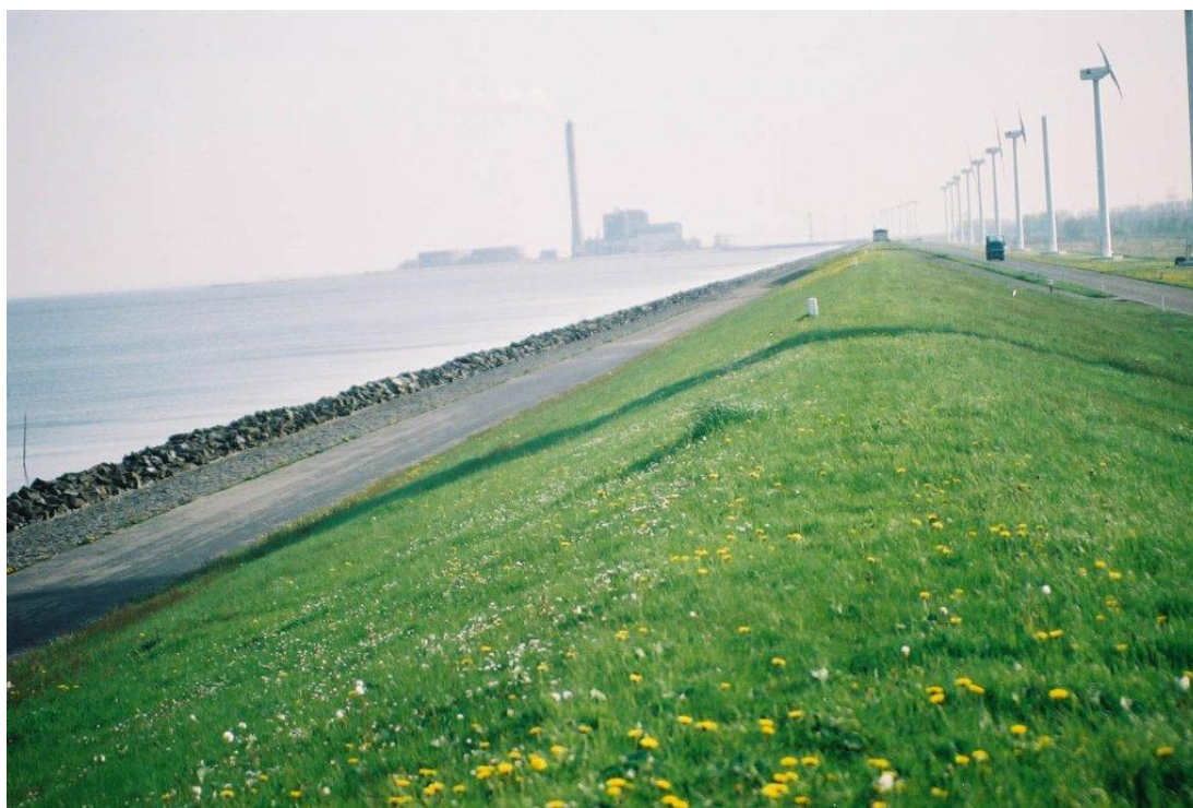
Figure 2.20. Dike along Flevoland near the power plant, facing the IJsselmeer.
