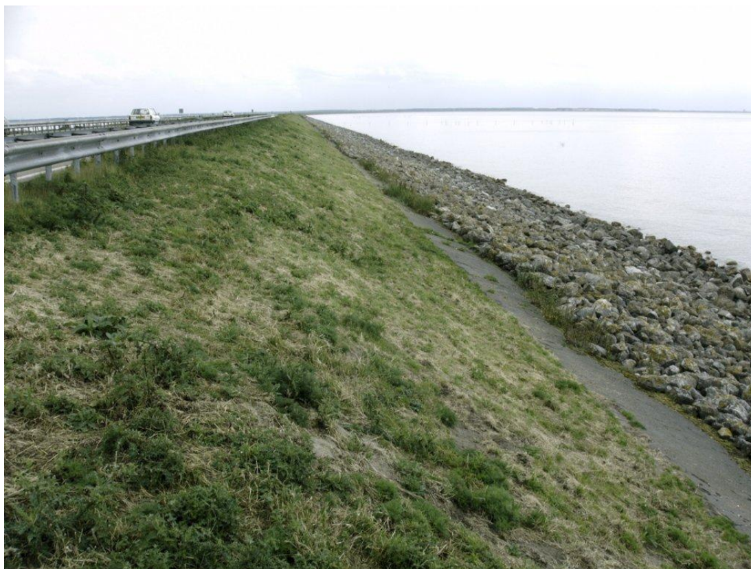
Figure 2.22. South side of Houtribdijk, facing the Markermeer.
