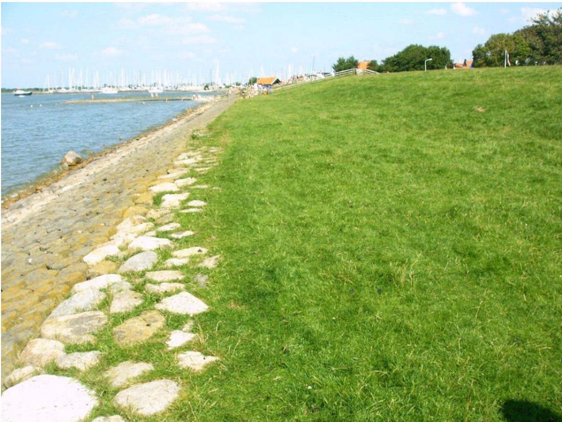
Figure 2.23. Dike in Friesland, facing the IJsselmeer.
