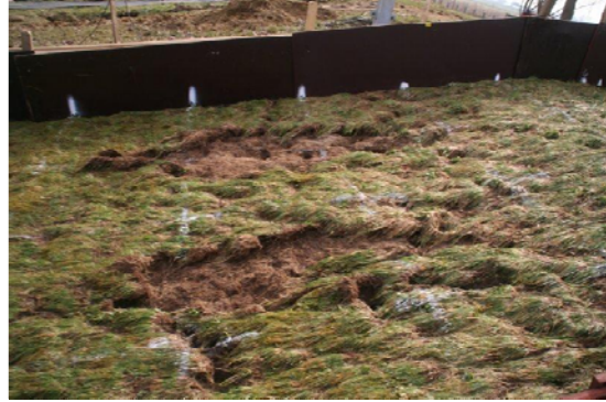
Figure 3.2. Various damaged locations
