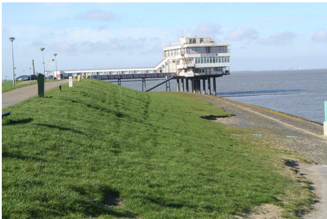
Figure 2.9. Seadike Groningen with the Eemshotel. Design water level 5.9 m +NAP; design wave height 1.2 m.
