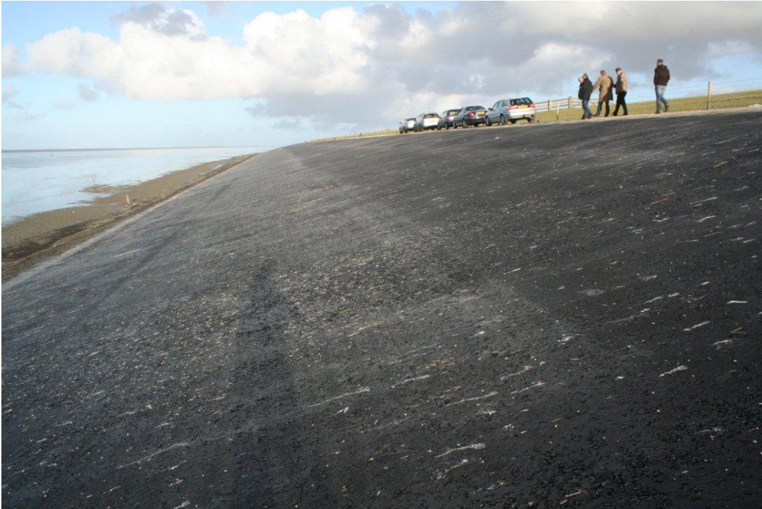
Figure 2.4. Boonweg - Waddensea. Seaward side, asphalt down slope 1:4.2.
