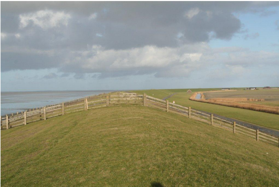
Figure 2.2. Boonweg - Waddensea. View from the crest. Landward slope on the right side. Upper grassed seaward slope 1:5.2.
