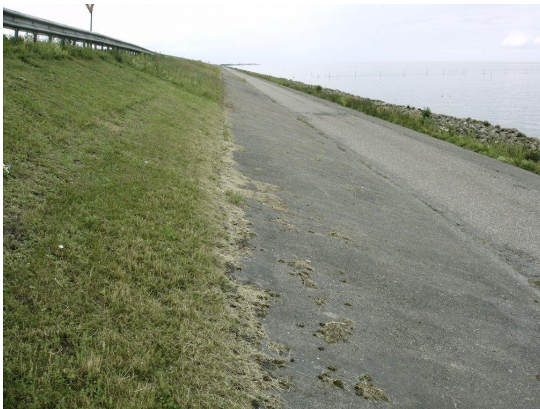
Figure 2.21. North side of Houtribdijk, facing the IJsselmeer.
