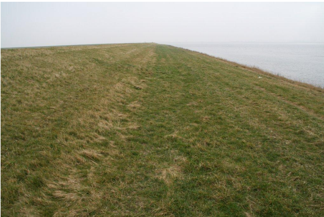
Figure 2.5. St Philipsland - Eastern Scheldt. Seaward side, upper grassed slope 1:3.5 with grassed berm 1:20.
