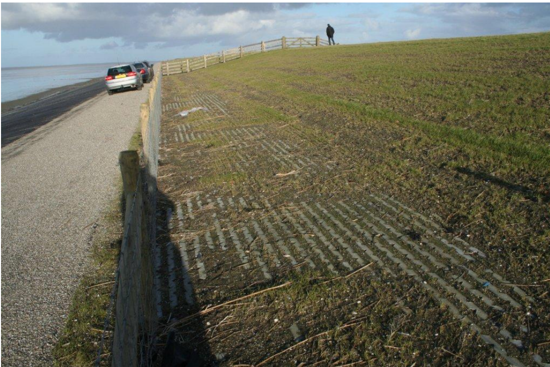
Figure 2.3. Boonweg - Waddensea. Seaward side, asphalt berm 1:7, open revetment 1:7 and 1:5.2 grassed upper slope. Berm between 6.3 and 7.3 +NAP.
